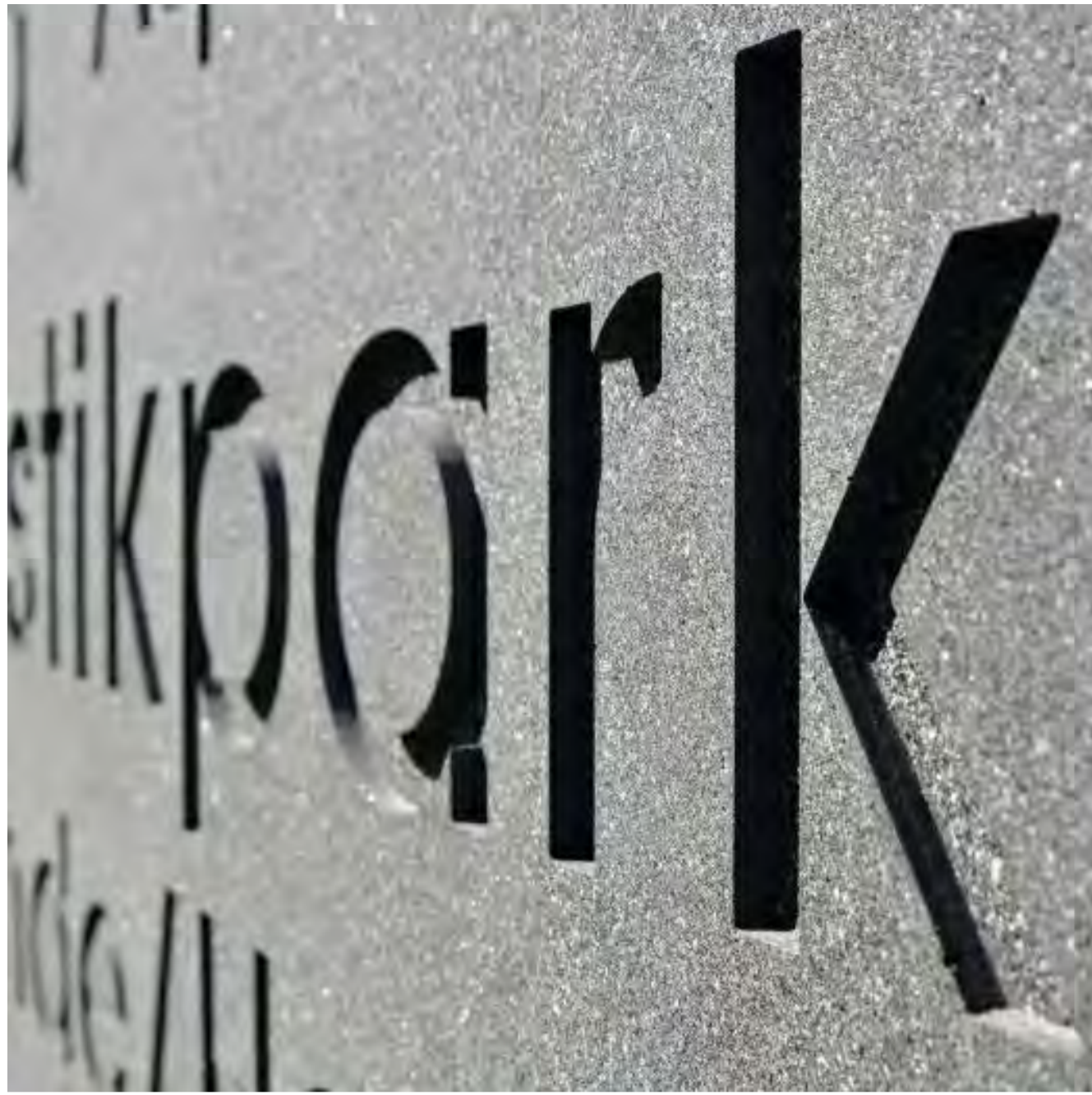
CUSTOM CONCRETE FORM LINER WITH 50MM PATTERN DEPTH OR SIMILAR. IMAGE INDICATIVE ONLY.
