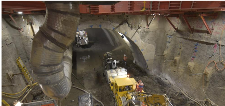
A'Beckett Street Shed, January 2019
