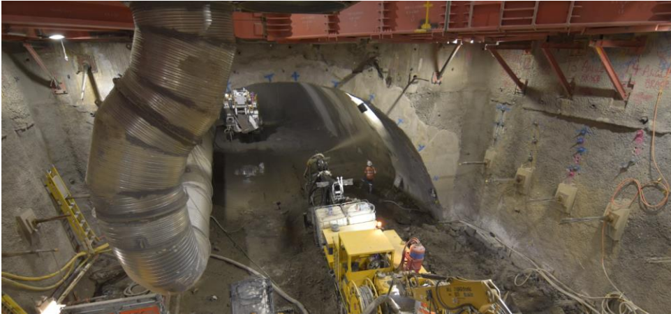
A'Beckett Street Shed, January 2019
