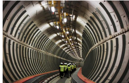
Example of tunnel boring machine tunnelling
