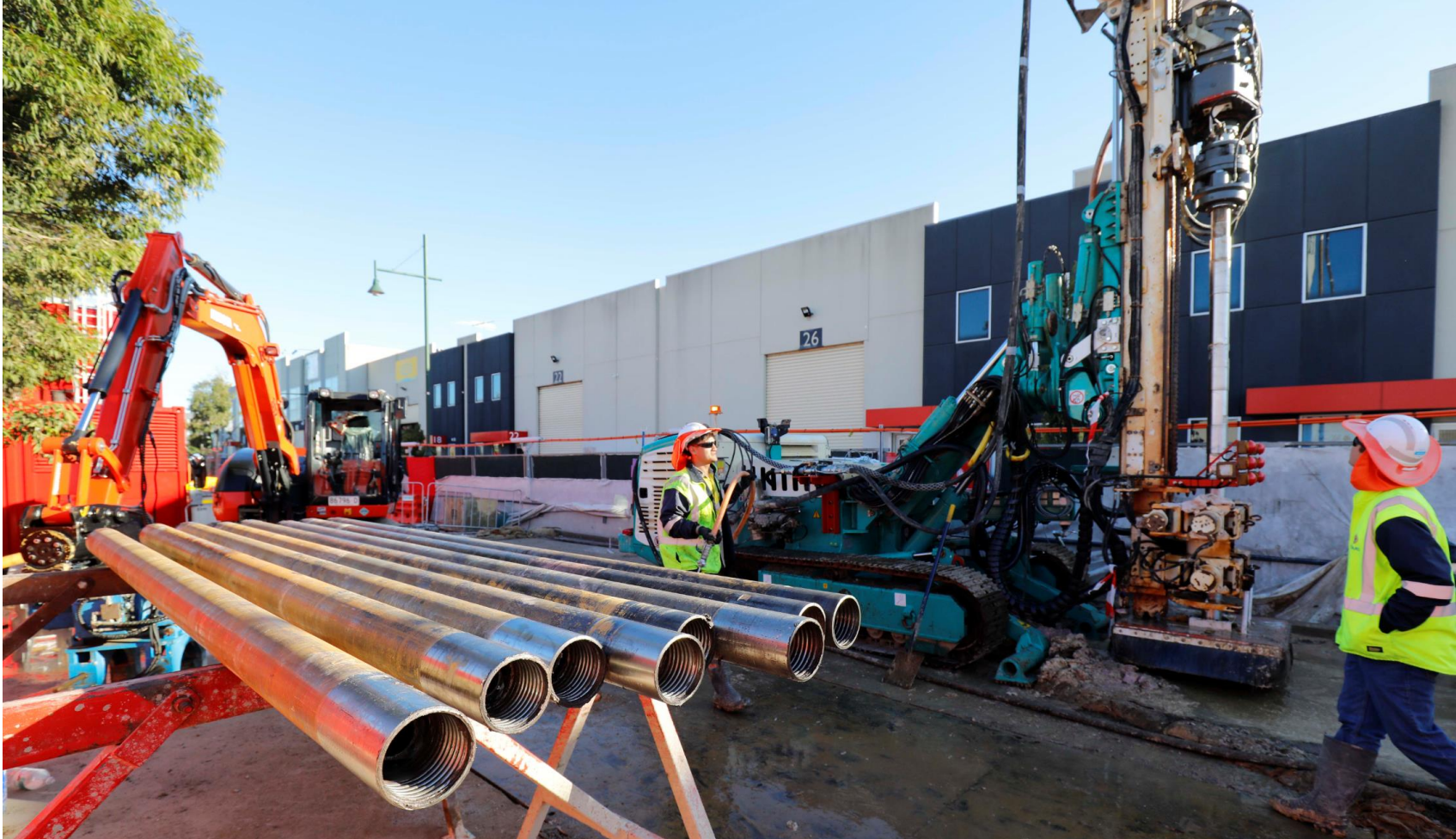
JET GROUTING SET UP – CROSS PASSAGE 2
