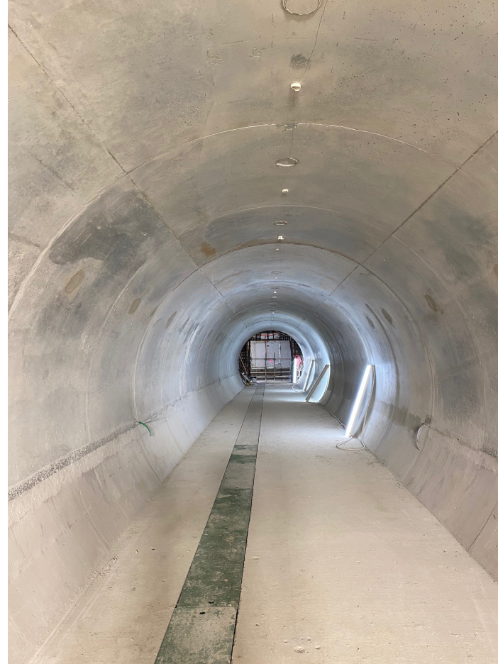
Permanent lining works complete (CP4)
