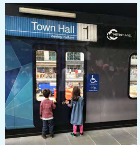
Viewing platform at City Square construction site.
