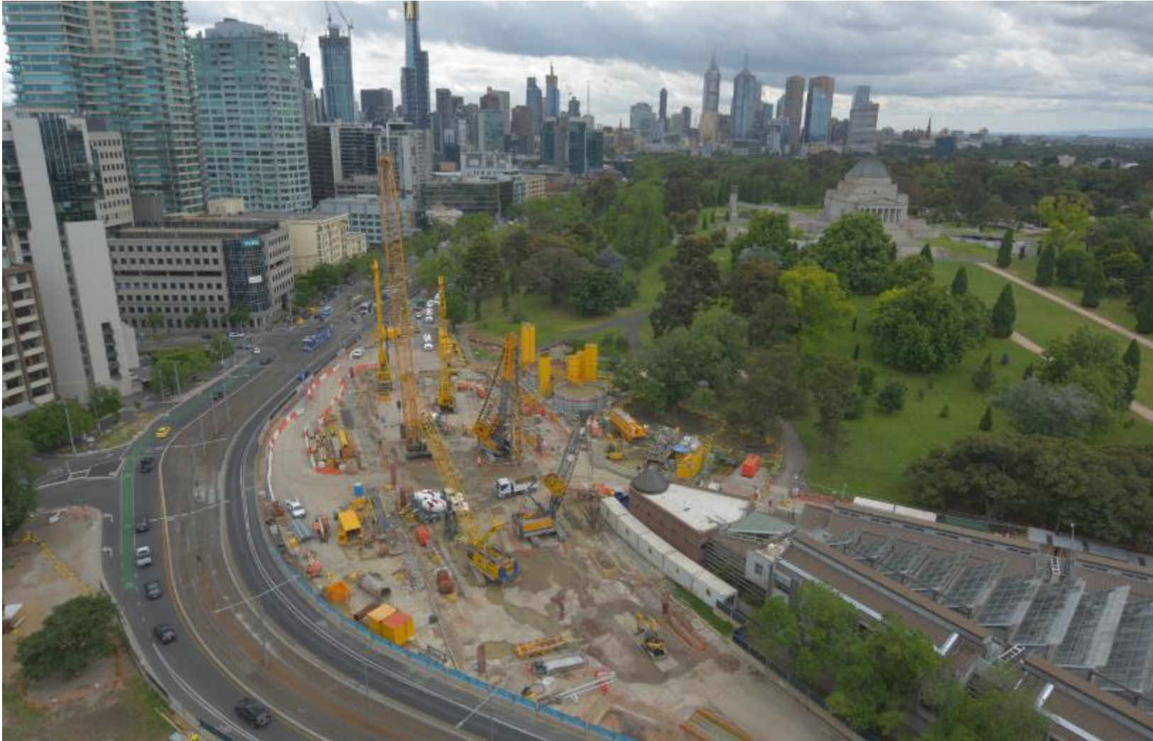
Timelapse image of northern station box works
