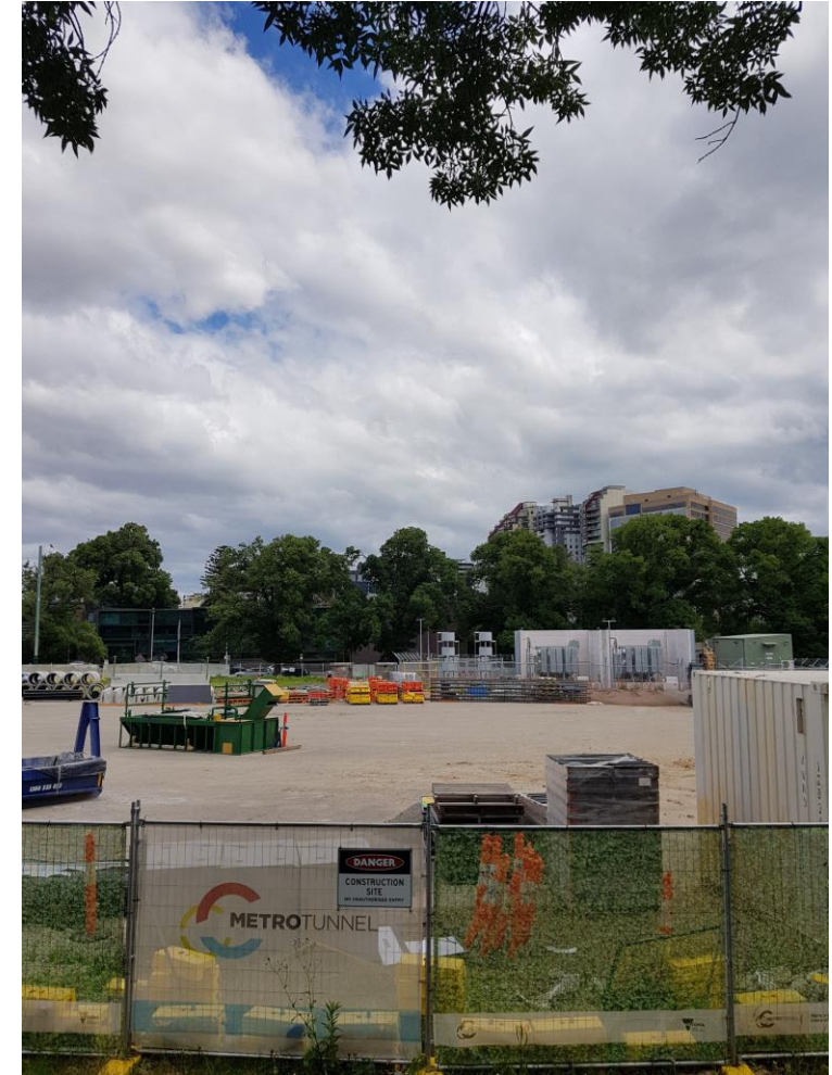
Tunnel Boring Support Site – Edmund Herring Oval
