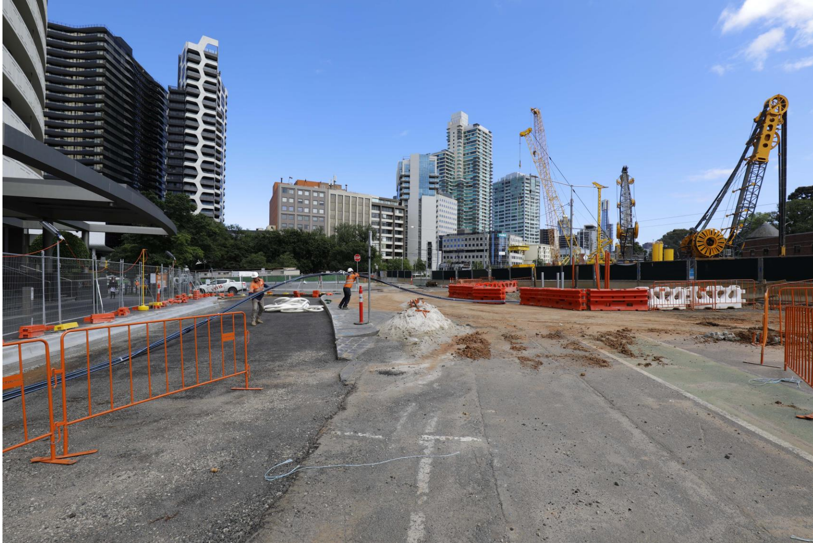
Construction underway of the new St Kilda Road service lane between Bowen Lane and Albert Road
