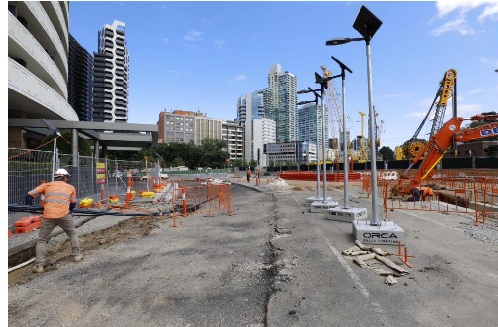
South Box road works
