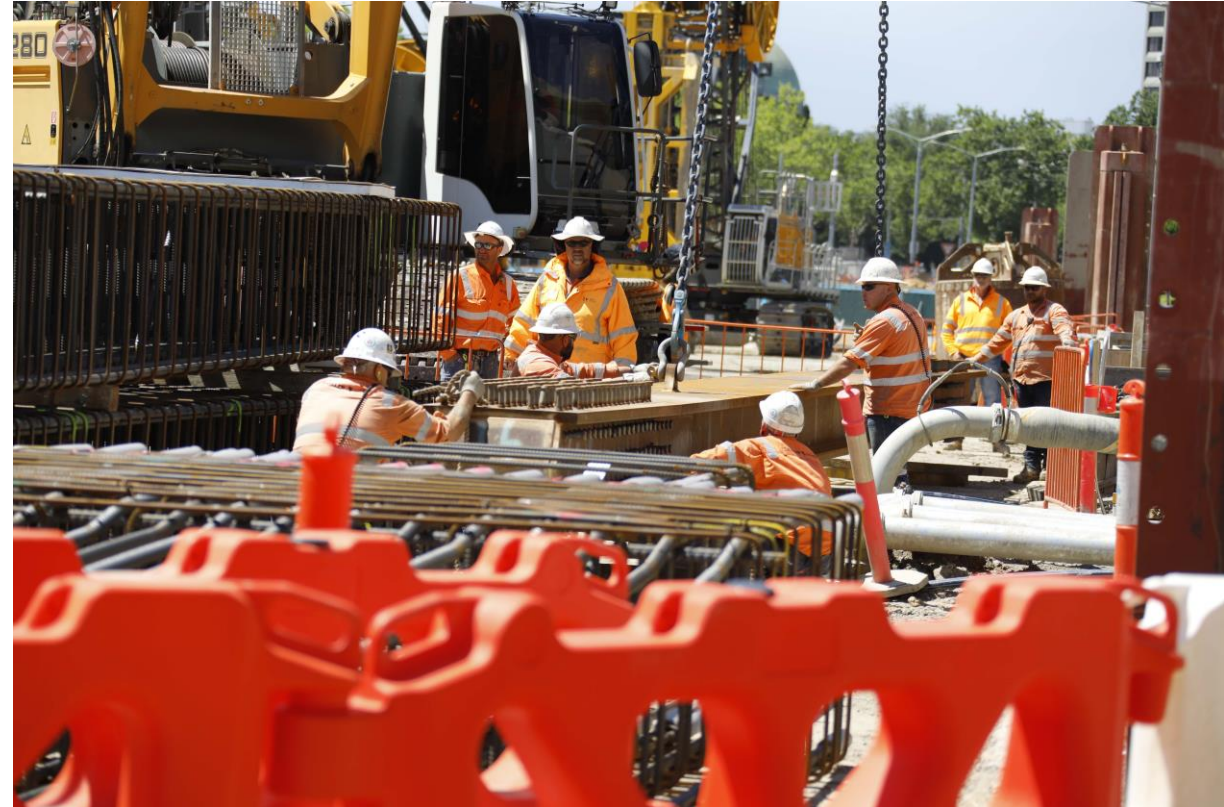
Northern section D-Wall works
