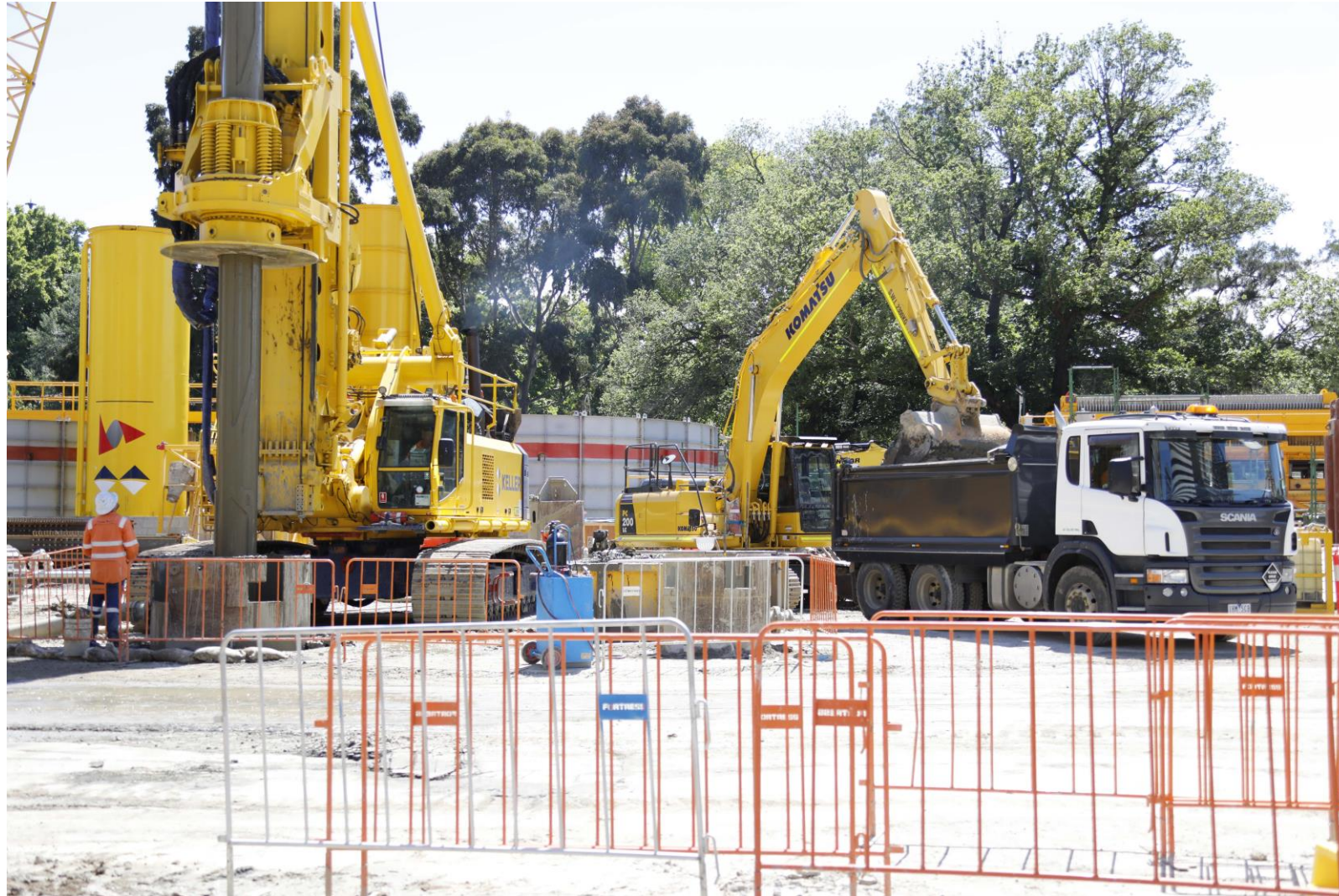
Northern section central piling works
