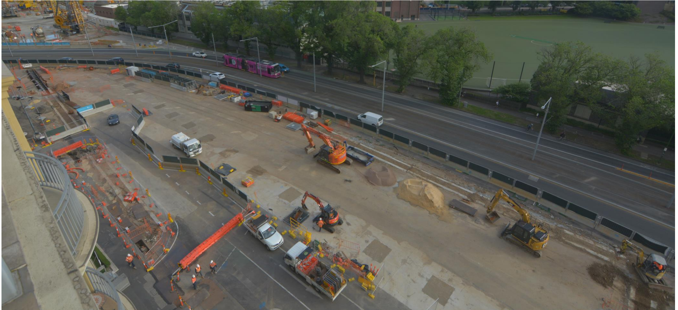
Timelapse image of southern station box works
