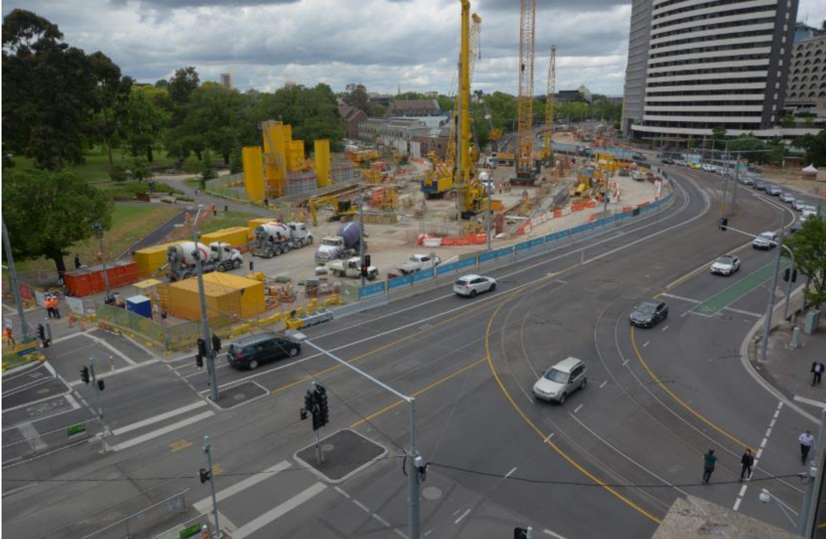
Timelapse image of north section station box works
