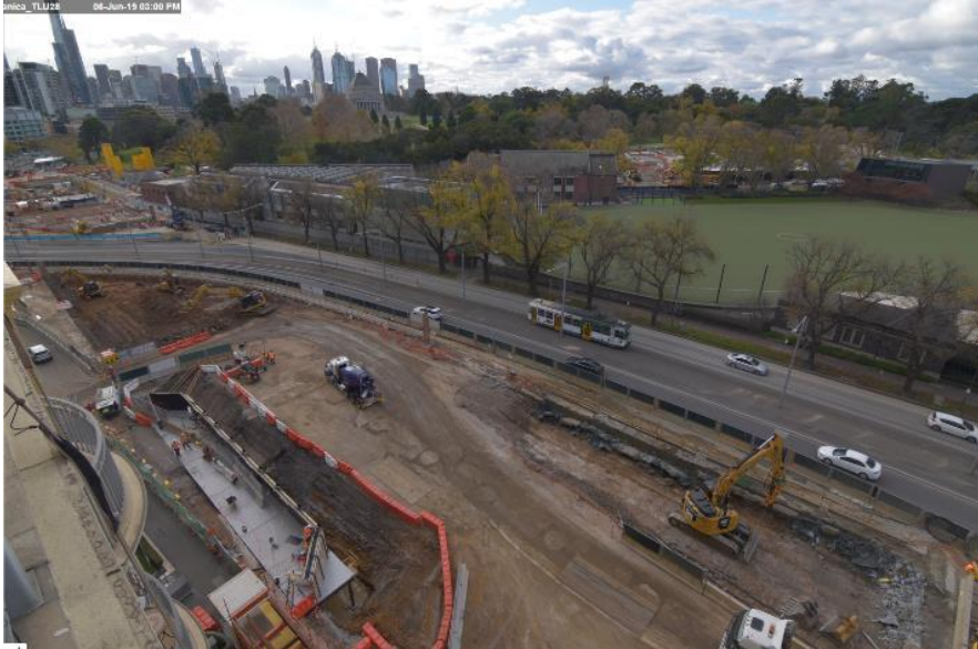
D-wall breakout during south box roof construction
