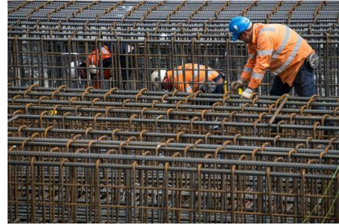
Steel tying works in the north box
