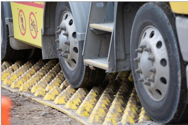
The Metro Tunnel Project continues to explore new and innovative ways to reduce the impact of construction activities on the local community. Recently we have been trialling a new type of ‘rumble grid’ near our William Street entrance which is designed to shake excess mud off vehicle tyres and help us reduce the dirt on nearby roads.
