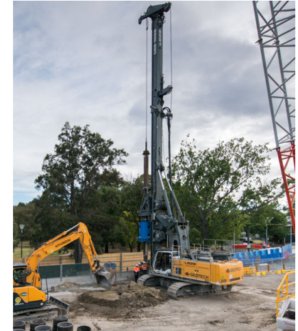
Piling machinery used to construct the TBM Retrieval Shaft
