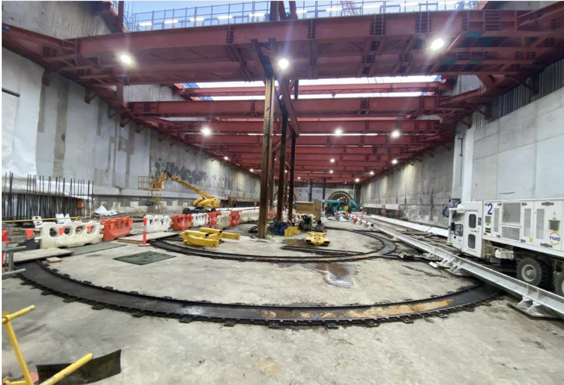
TBM gantry retrieval rotational device
