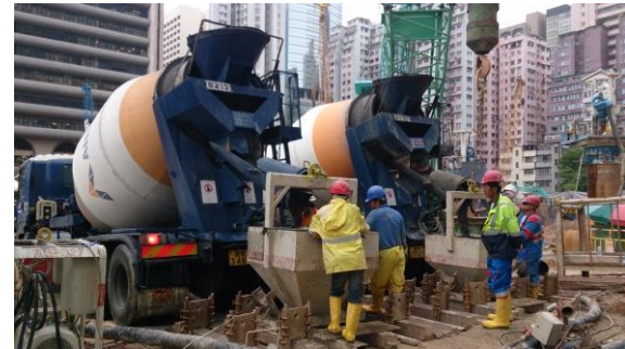
Placing reinforcement and concreting
