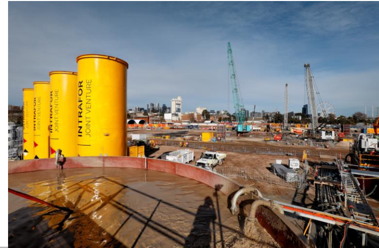
Bentonite plant at Arden site
