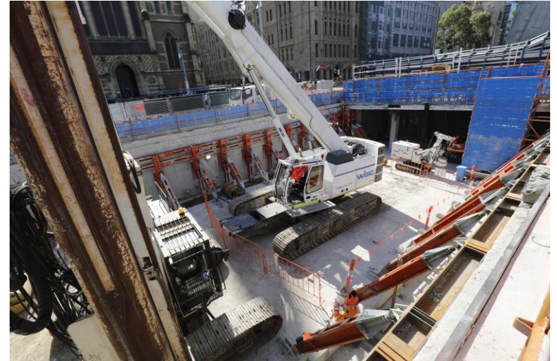
APRIL- JULY PILING
