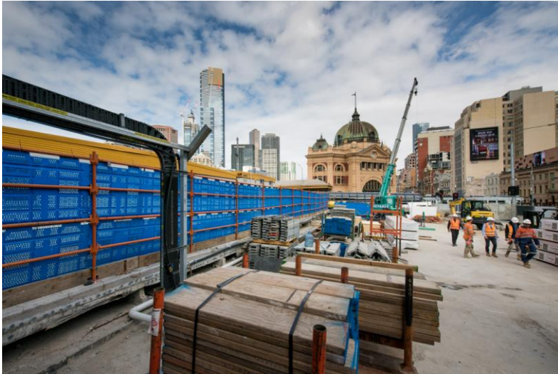
MARCH- DEMOLITION COMPLETION
