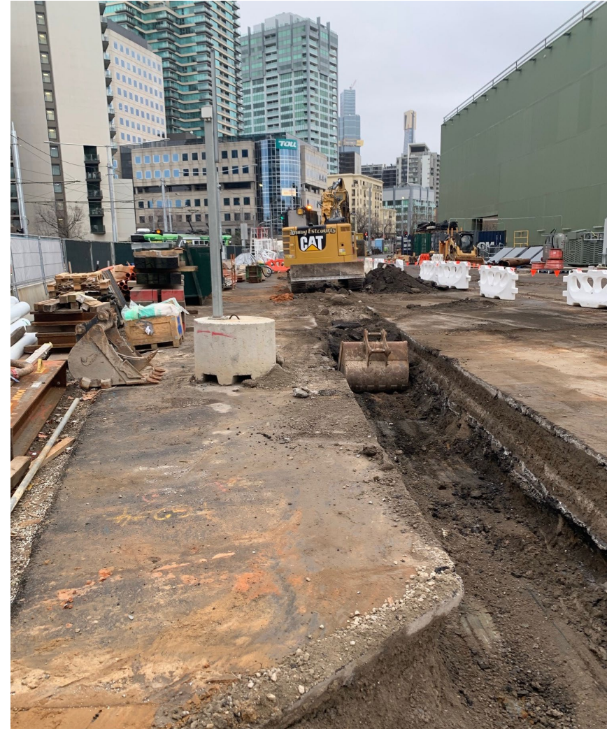
Obstruction Removal ahead of piling
