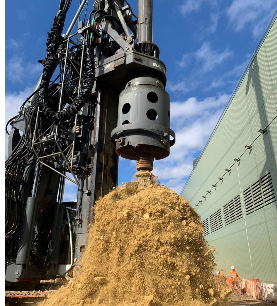
Piling works underway at the station entrance
