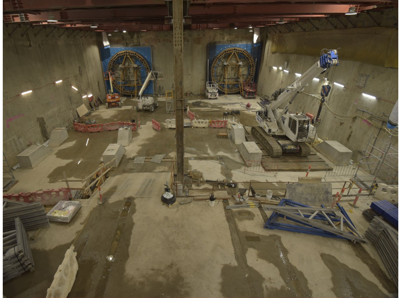
The construction of the north headwall
