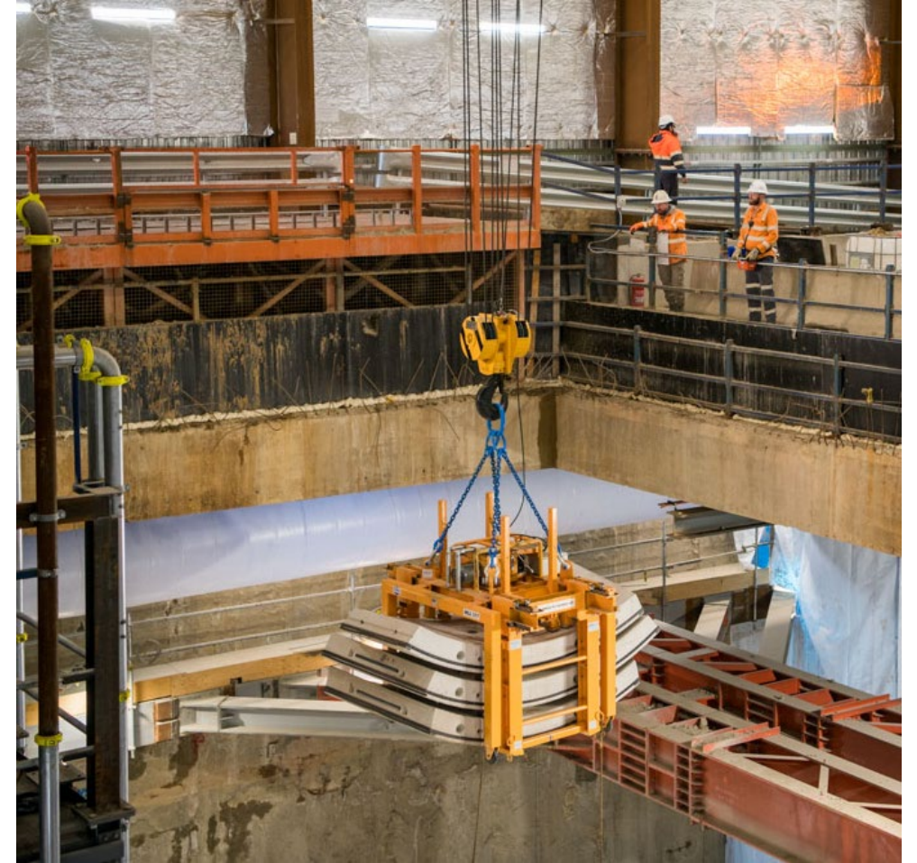
Concrete segments being lowered to the TBM
