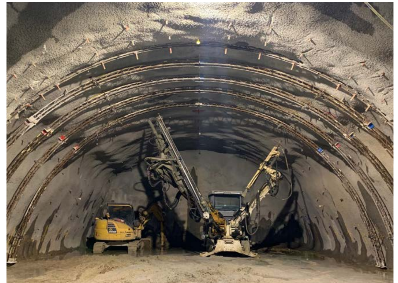
Town Hall Station's central cavern takes shape under Swanston Street.
