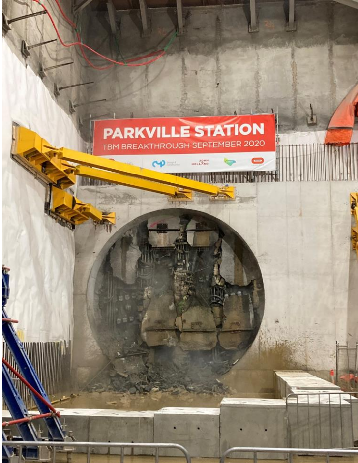
Breakthrough process ongoing
