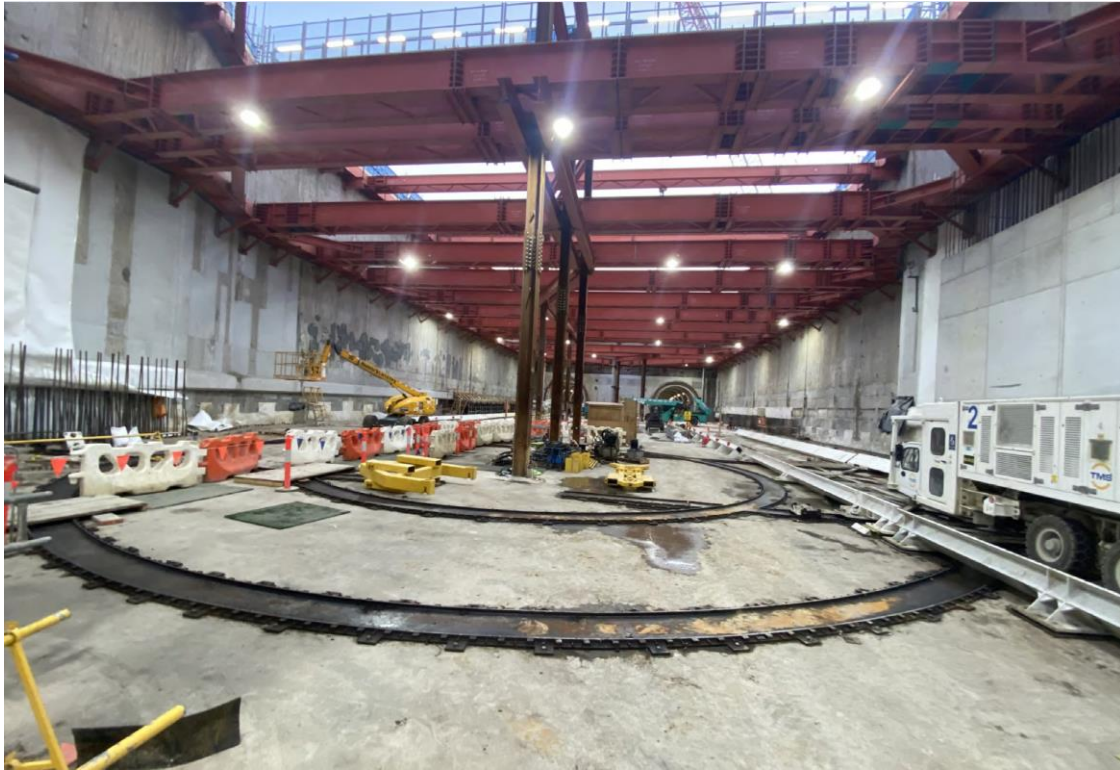
TBM gantry retrieval rotational device
