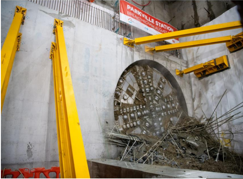
Breakthrough process ongoing
