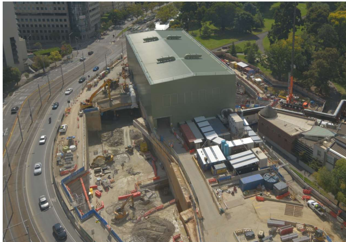
Excavation of pits and conduit trenches in the tram interchange
