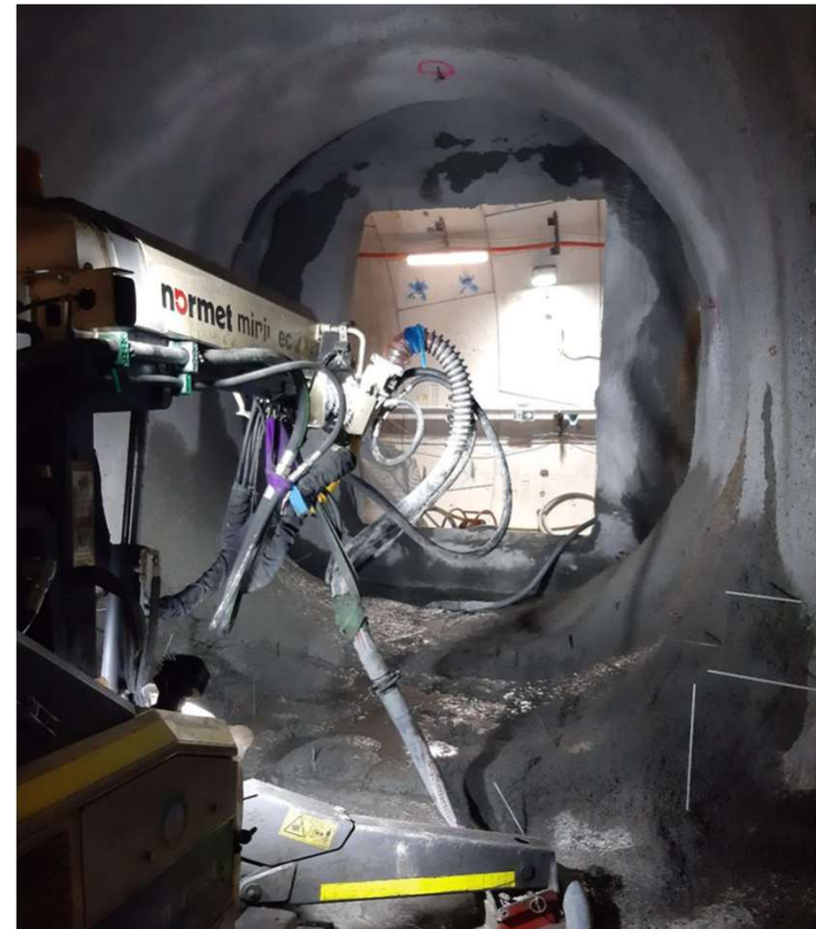
Shotcreting cross passage excavation
