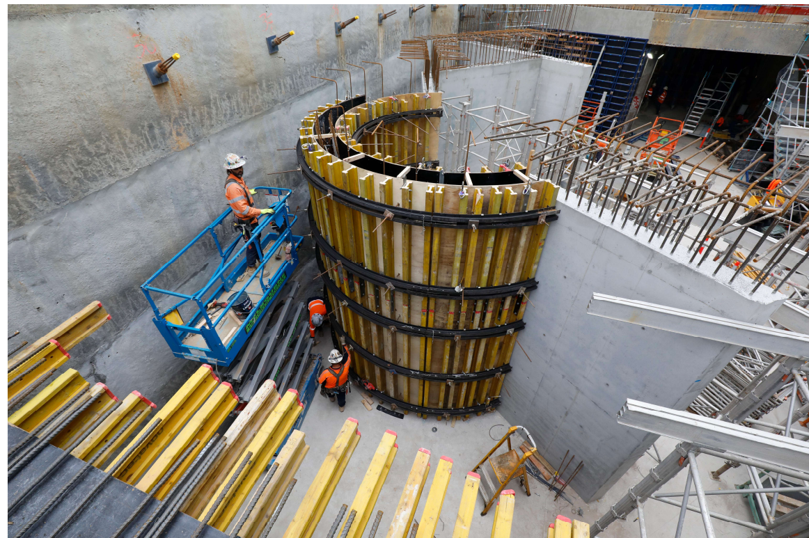
The lift well in the Shrine entrance prior to the final roof pour
