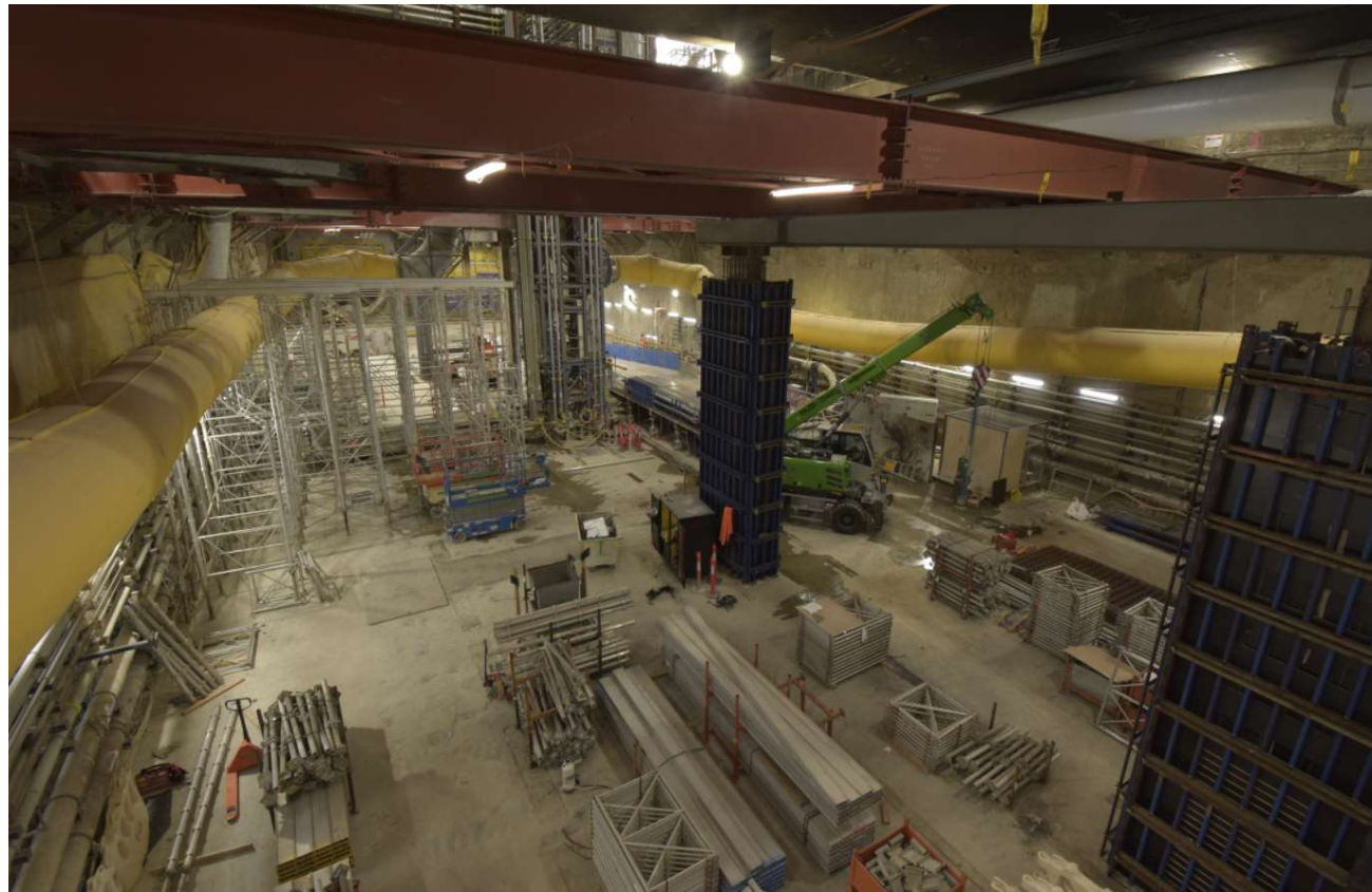
Start of falsework installation in the north box with formwork for internal columns
