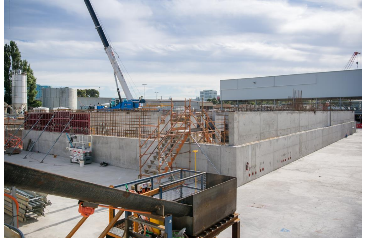
Construction of the services building upstand walls
