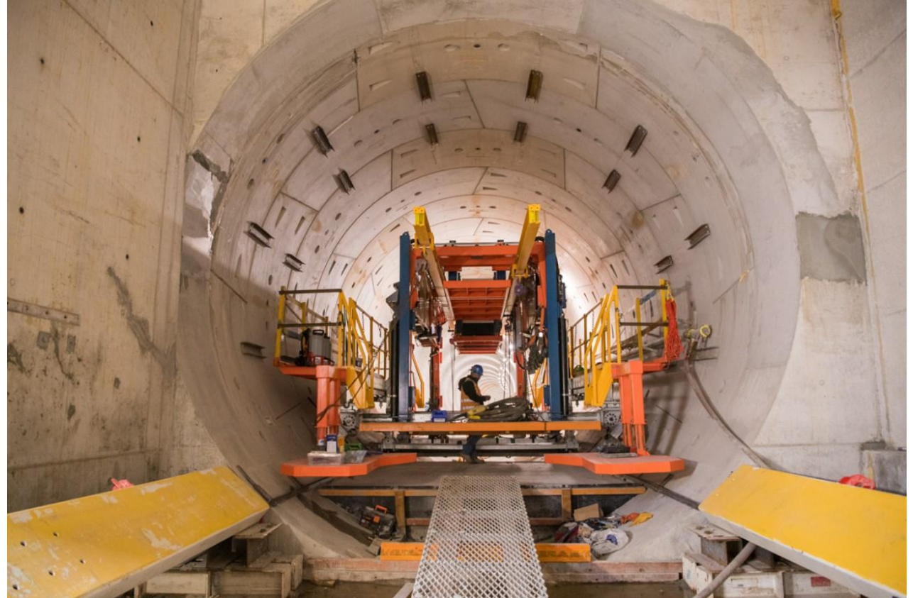
The screeding gantry used when pouring the tunnel invert
