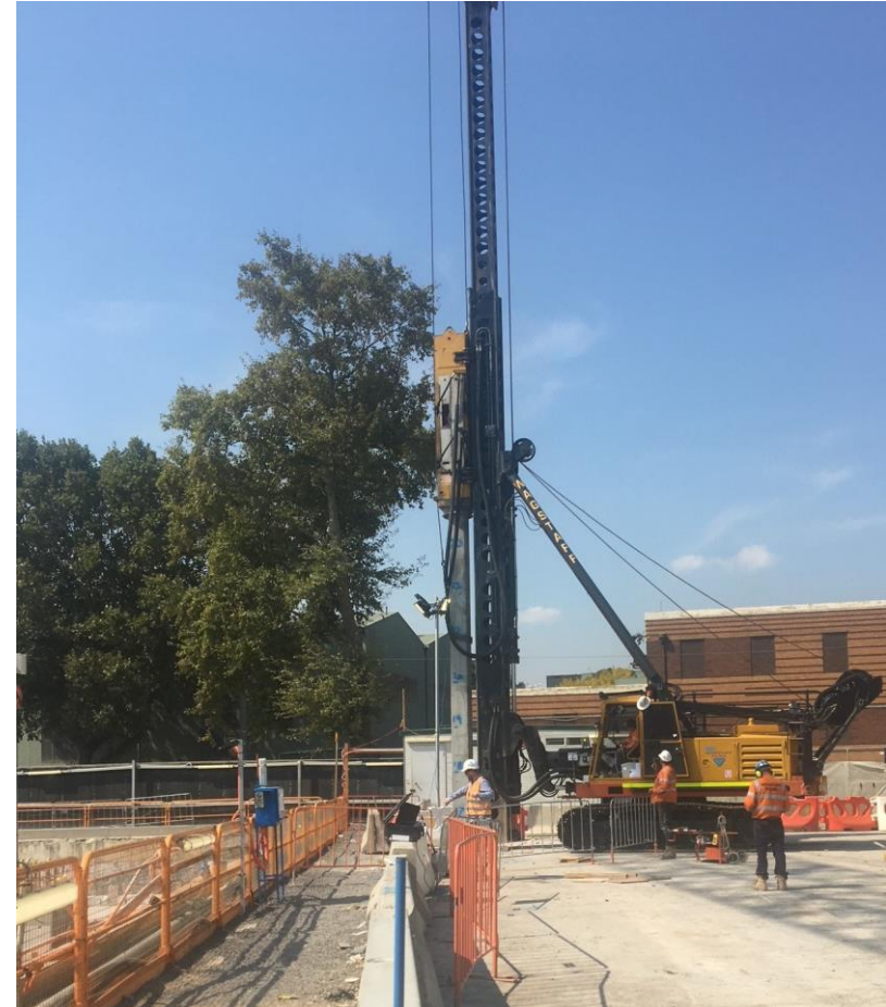
Driven piling underway in the south east corner of the station box
