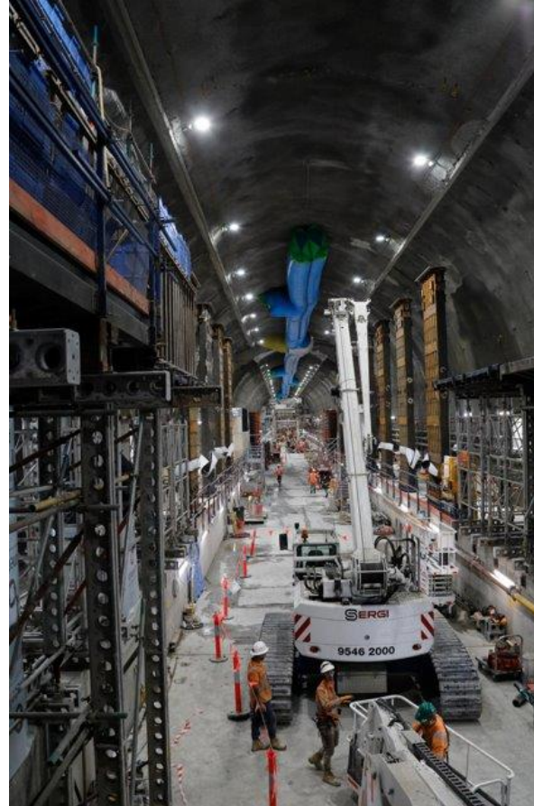
Structures and lining works within the central cavern
