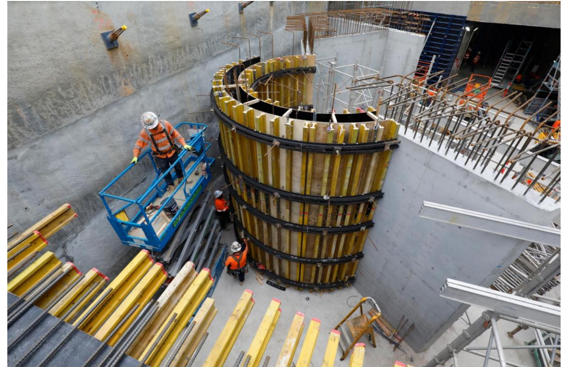
Shrine of Remembrance lift well falsework
