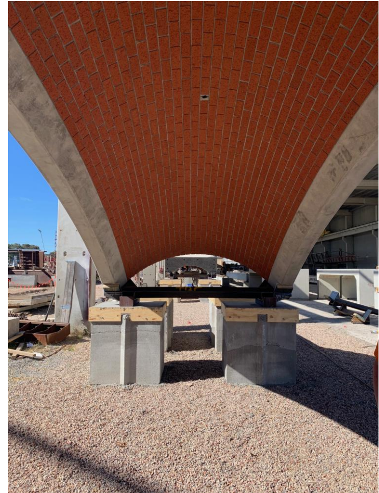
A pre-cast brick arch
