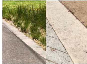
Sawn bluestone pitches and wide concrete edging
