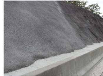
Shotcrete batters to rail corridor
