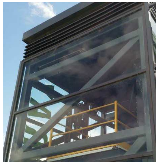
GLS-01 GLAZING PANEL TO LIFT SHAFT FACADE. PATTERN AND COLOUR SHOWN INDICATIVE ONLY
