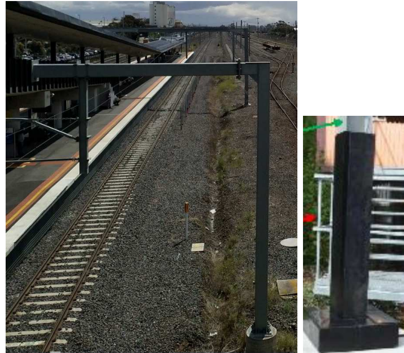
OVERHEAD WIRE TYPICALLY STEEL COLUMN (PAINTED/ GALVANISED) WITH 2400MM HDPE CLADDING ABOVE FLOOR LEVEL, PAINTED IN BLACK
