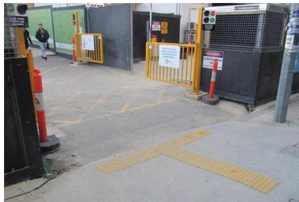
Image of gates installed at Metro Tunnel Site Parkville
