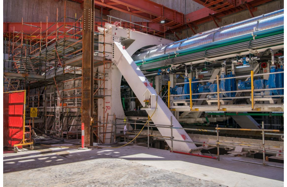
TBM Meg commissioning
