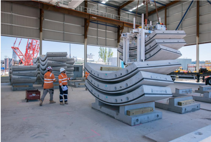
Pre-cast tunnel segments being delivered to site
