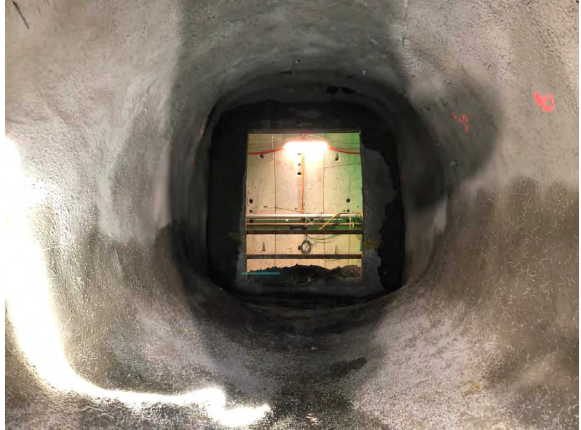
Cross passage lining finishing works – cross passage 2 (McLennan Drive)
