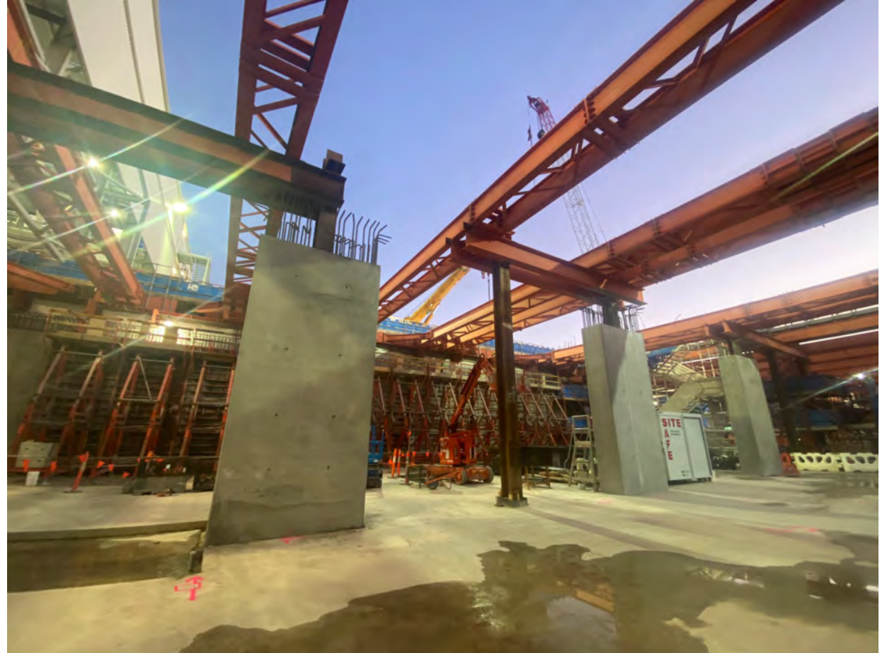
Completed rectangular columns (west box)
