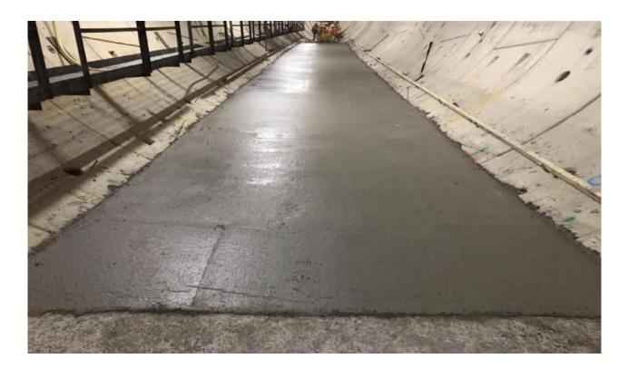
A section of first stage concrete invert works in eastbound tunnel
