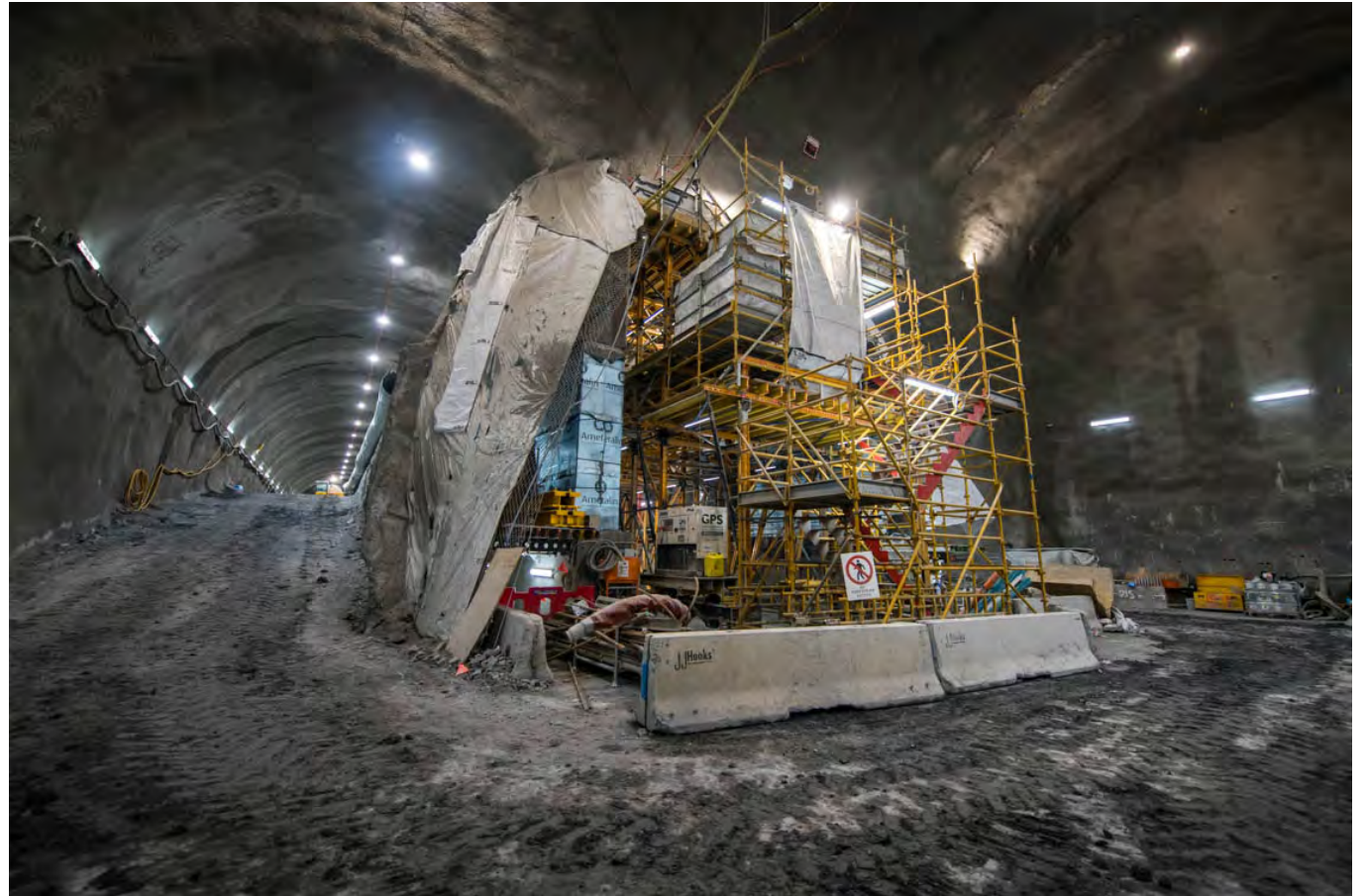
Excavation of the rail tunnels adjacent to the central cavern -
