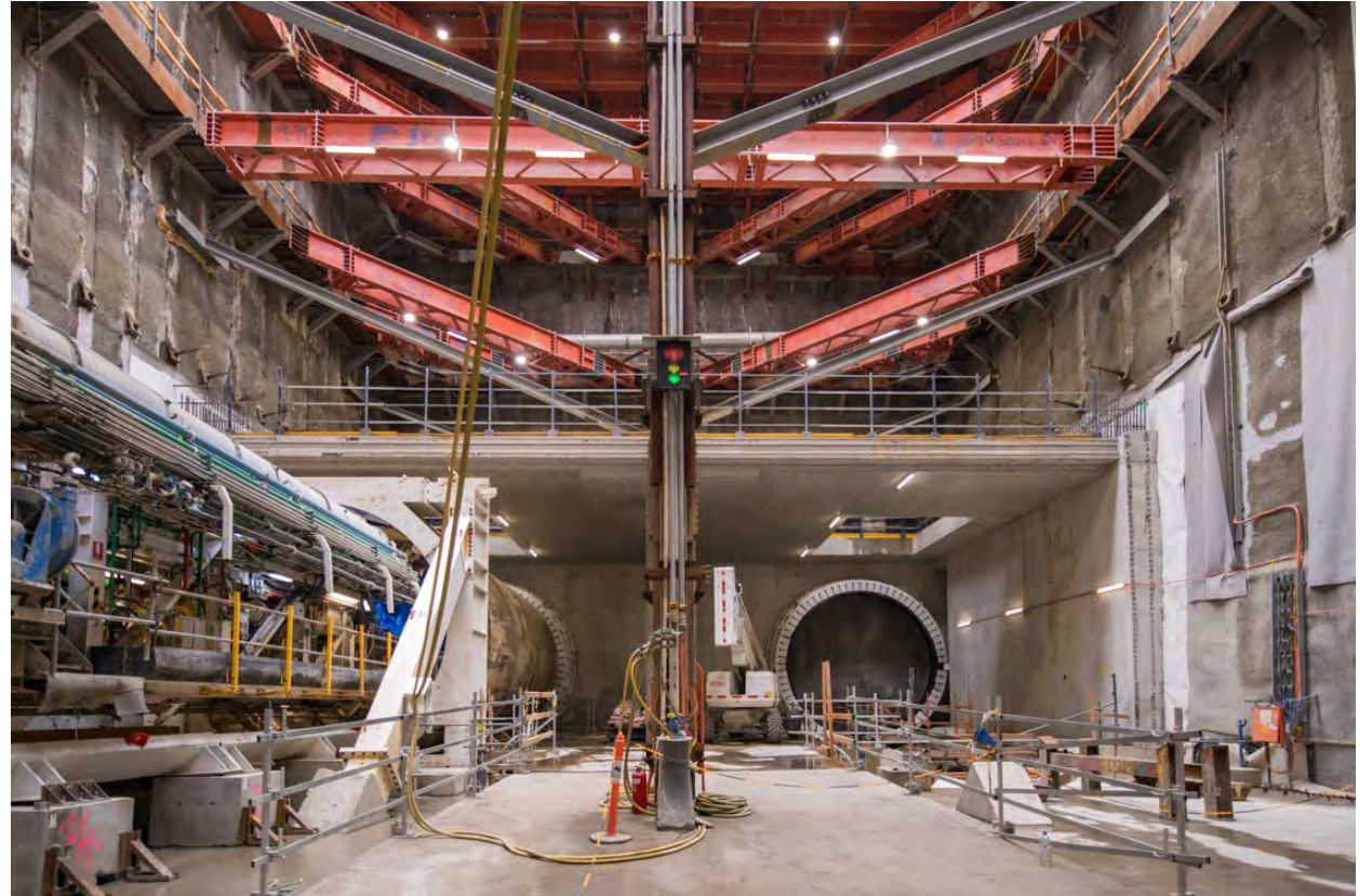
TBM 1 relaunch frame at the eastern end of the Grattan Street east site
