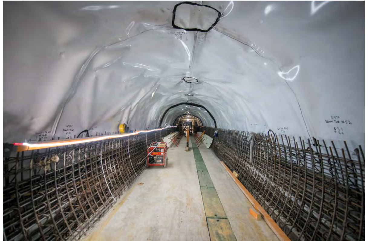
Cross passage waterproofing and invert (floor slab) complete
