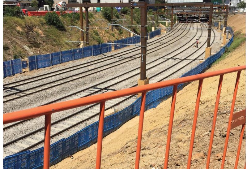
View towards Chapel Street from William Street Bridge
