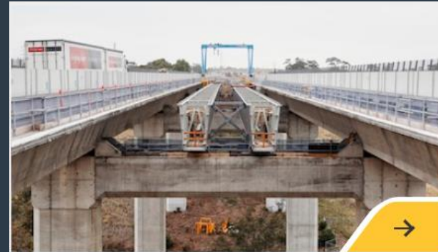
M80 Ring Road Upgrade
