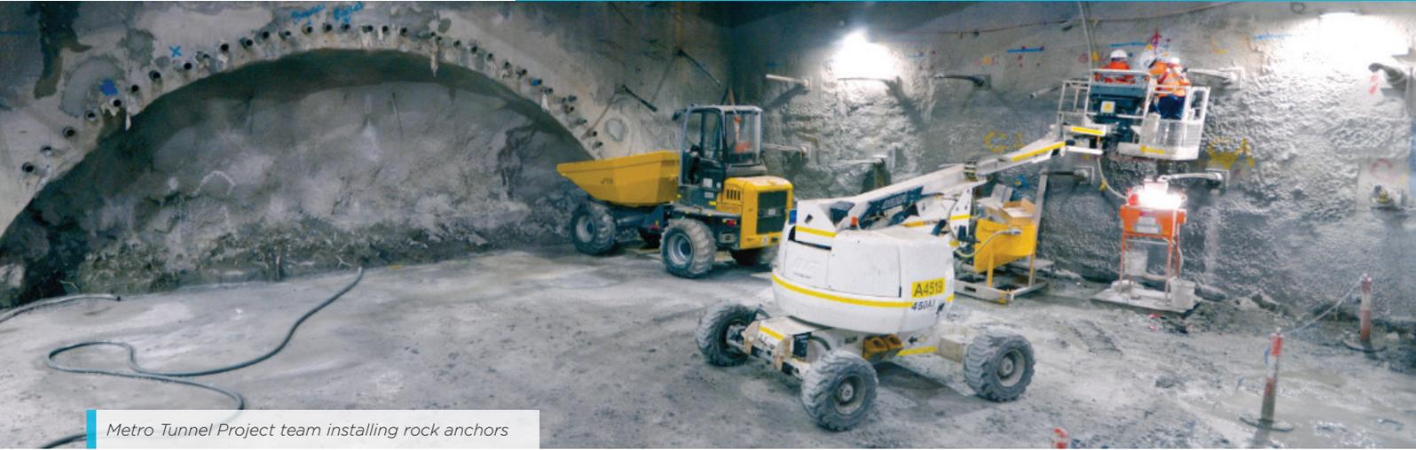
Metro Tunnel Project team installing rock anchors
