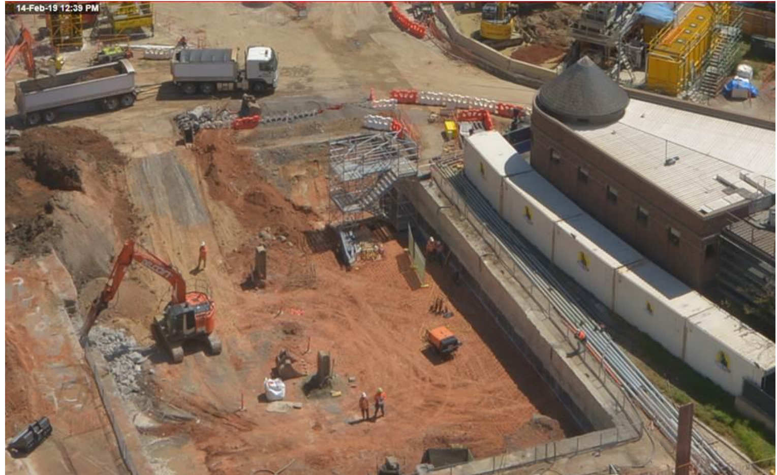
Works in the northern box
