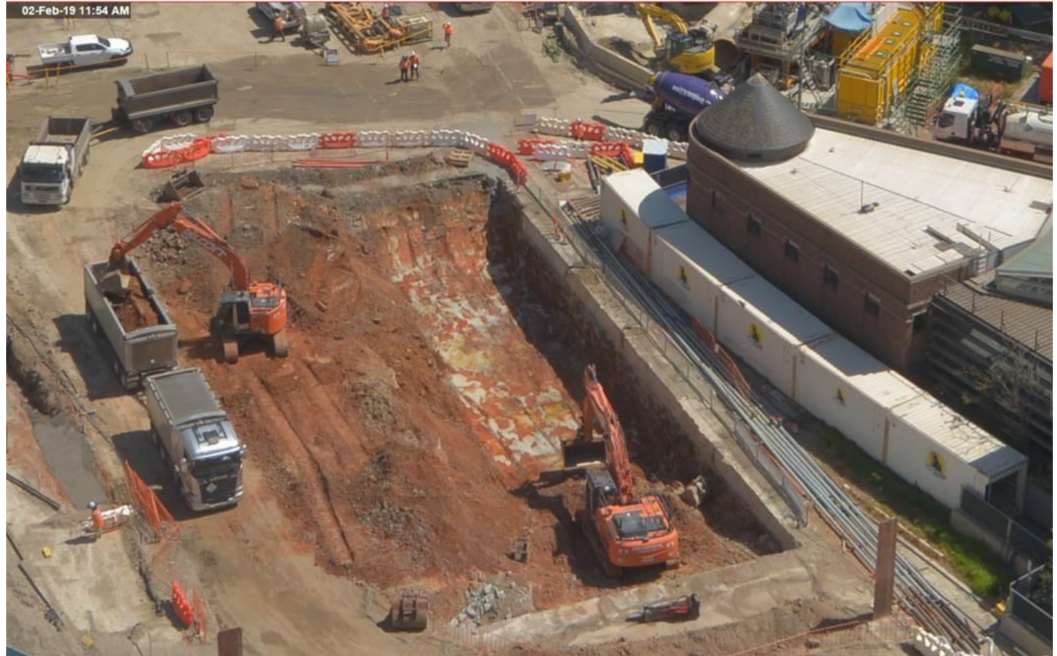
Works in the northern box
