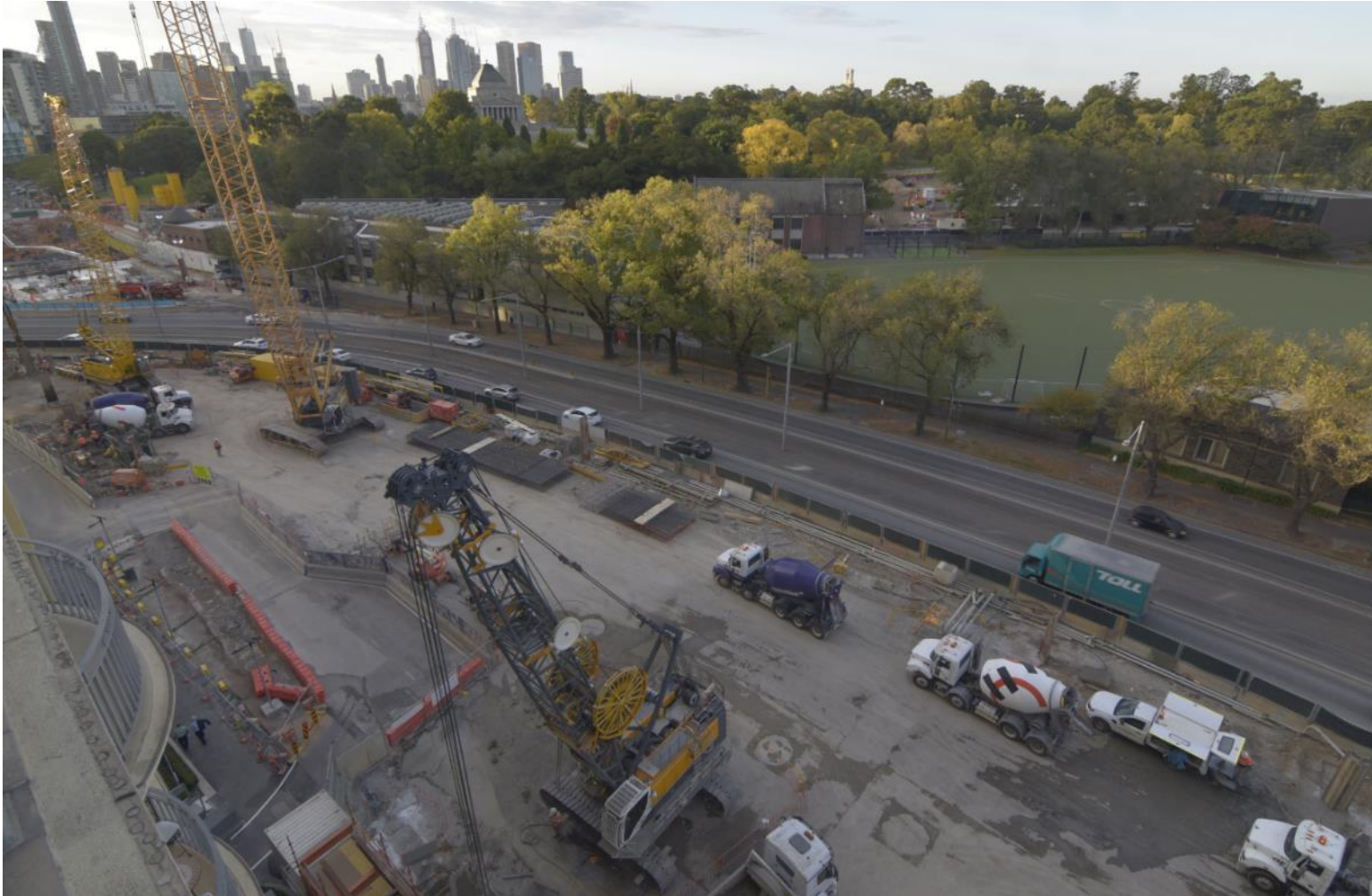
Timelapse image of southern station box works
