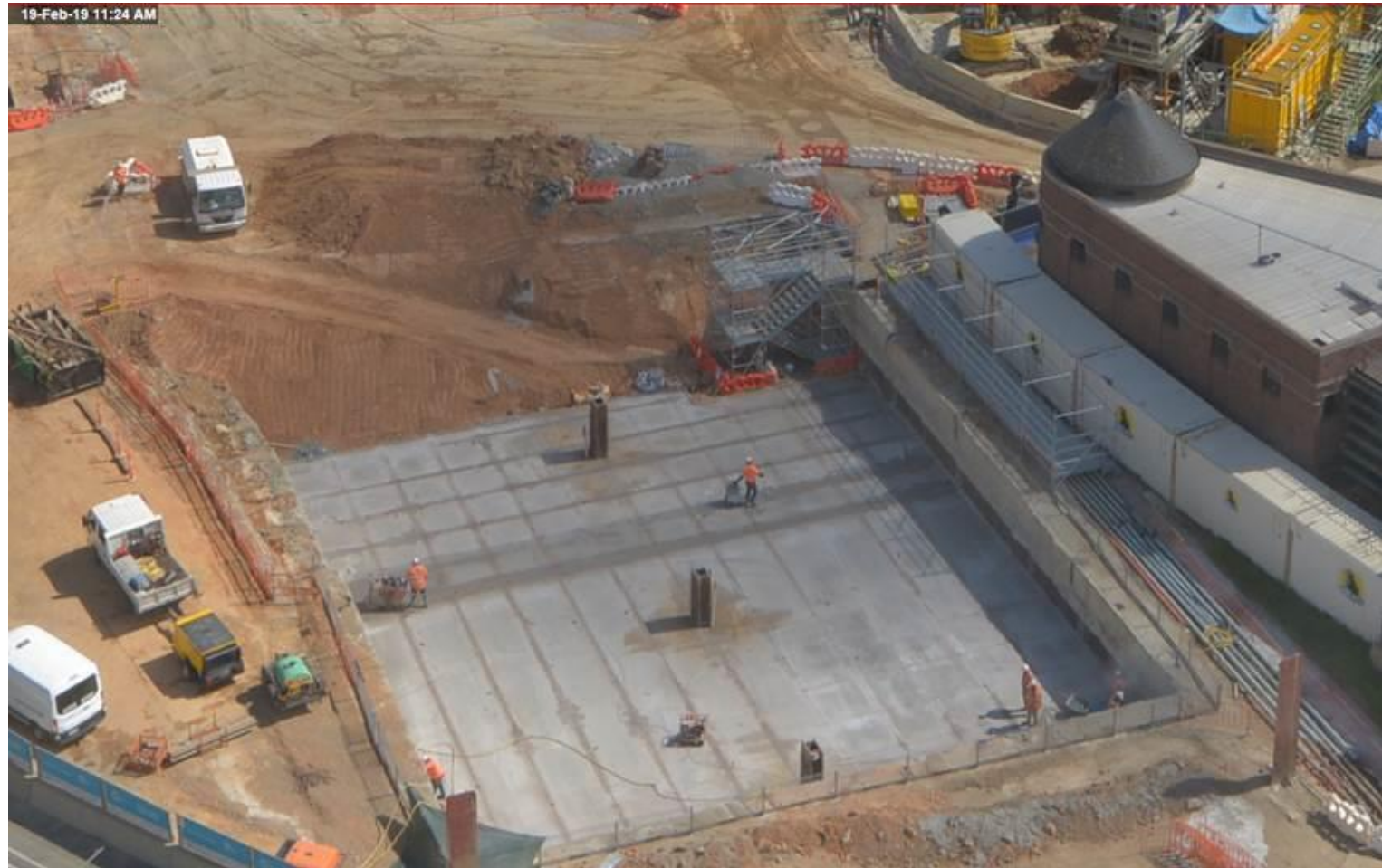
Works in the northern box
