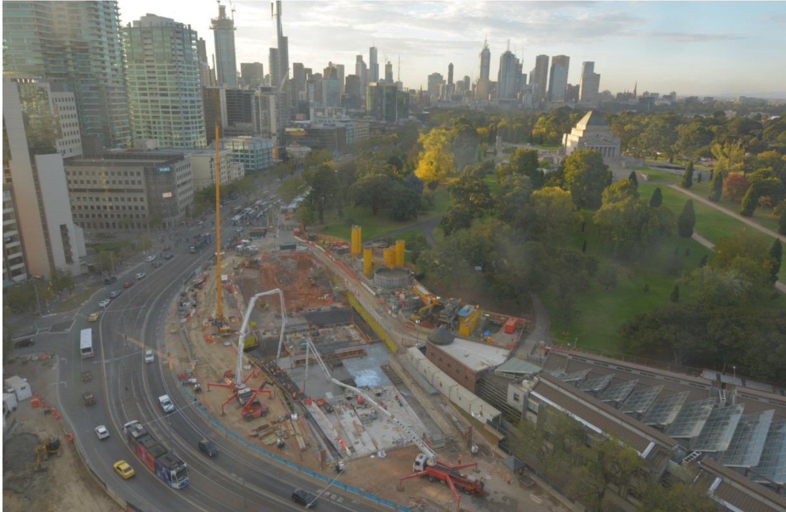
Timelapse image of northern station box works
