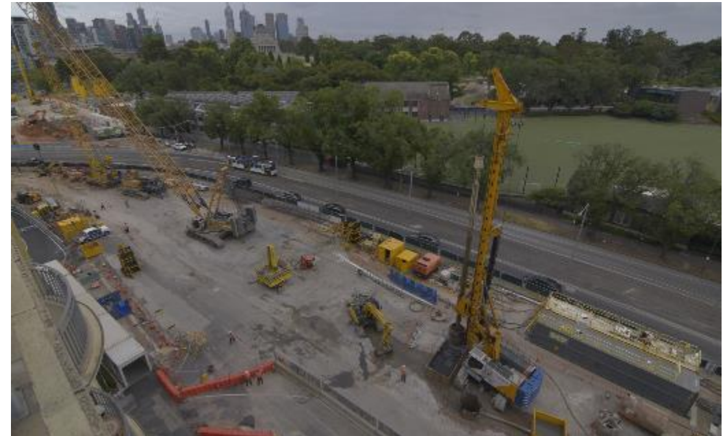
Southern section of works
