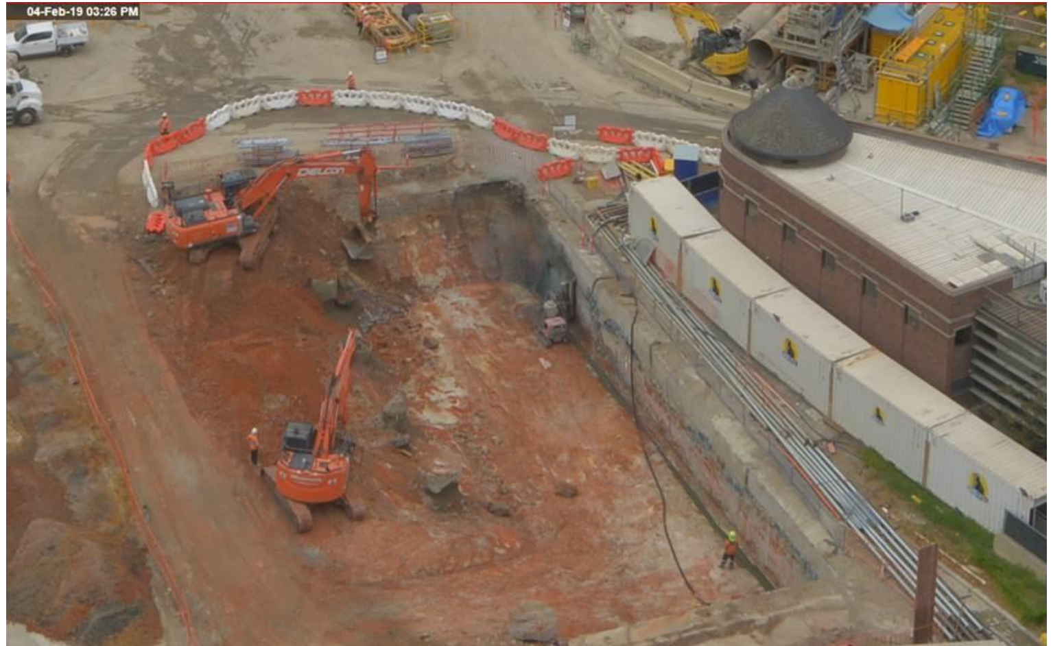
Works in the northern box
