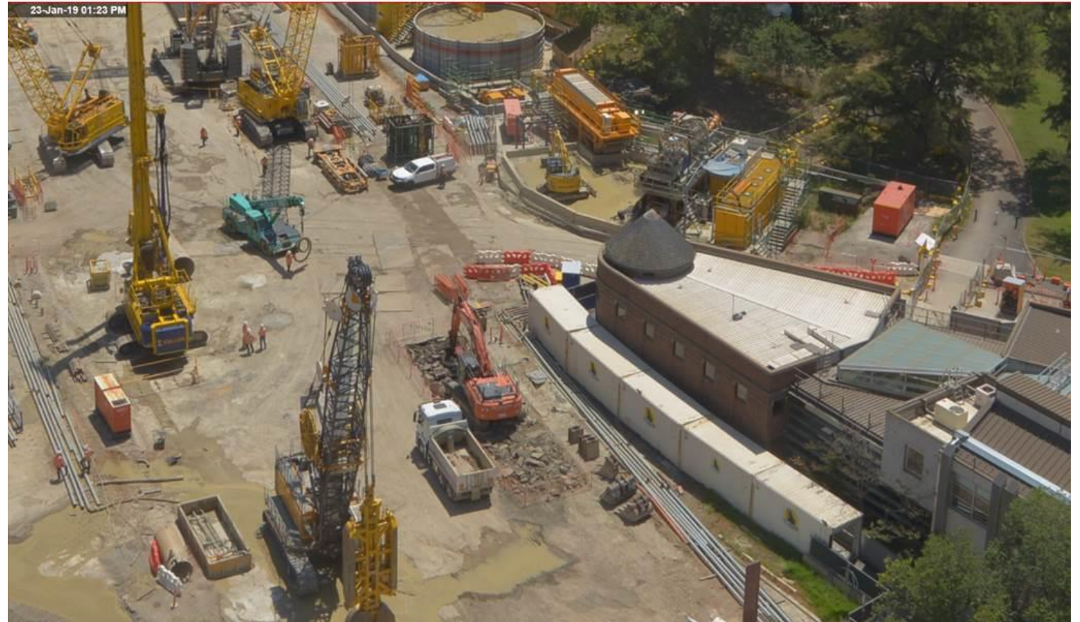
Works in the northern box
