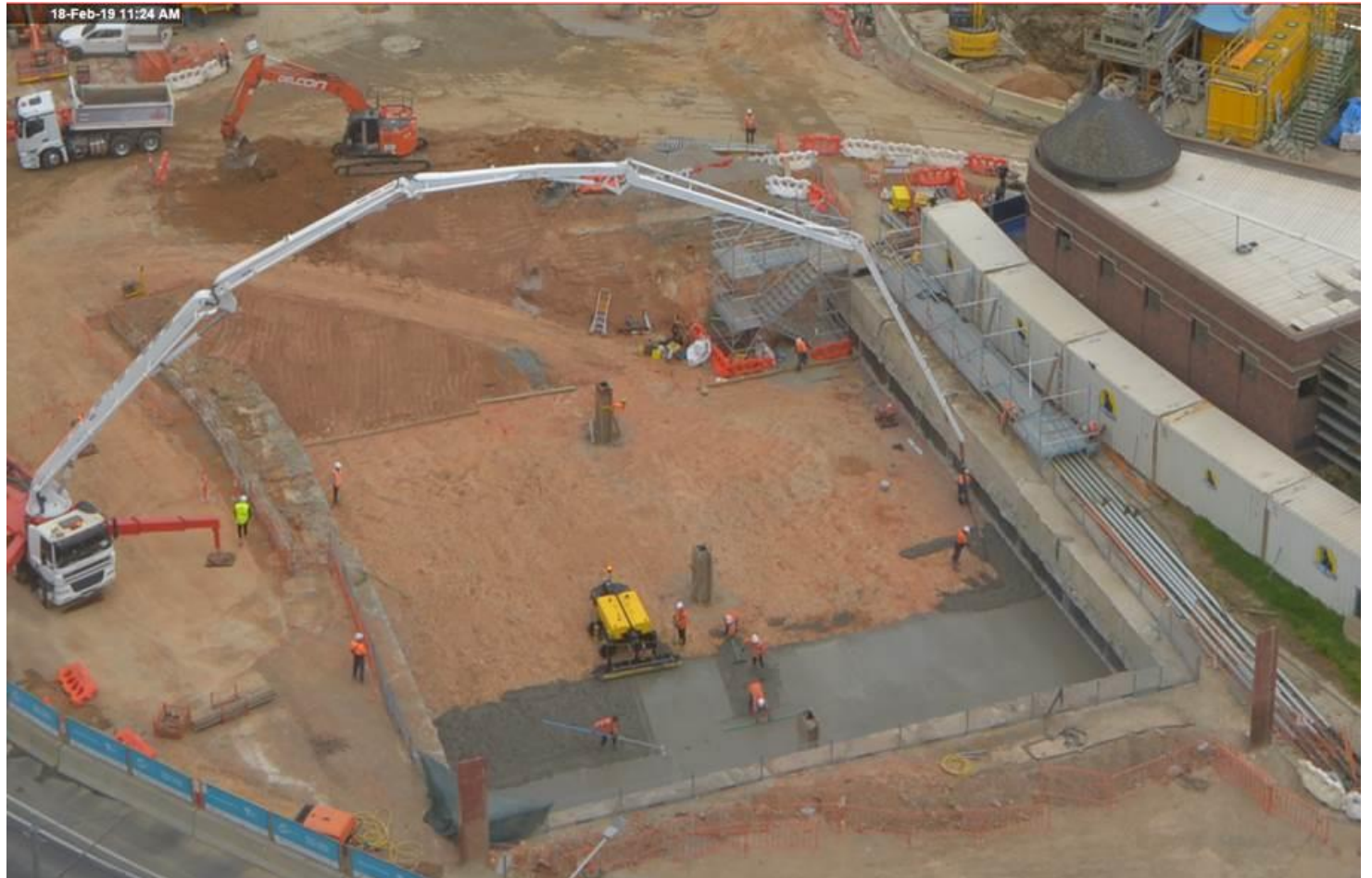
Works in the northern box
