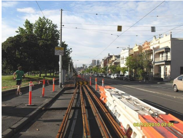
1. Pre-weld works – bringing rails in
