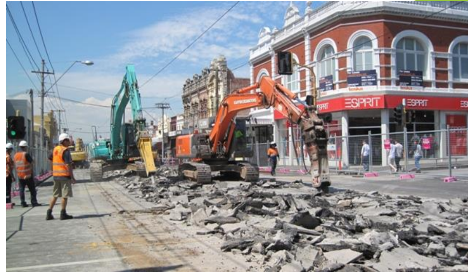
2. Breakout for excavation of existing tram tracks
