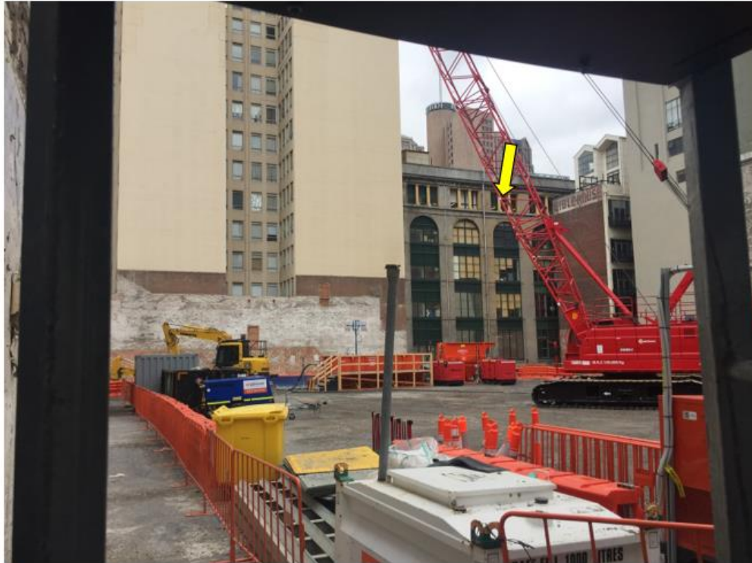
Noise monitor location at Ross House, Royston Place
