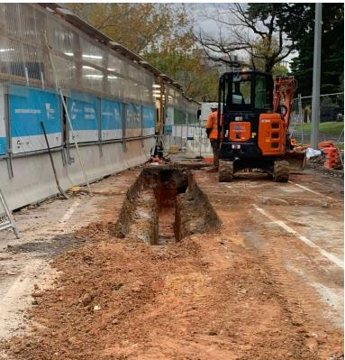
Trench excavation for relocated hydrant booster
