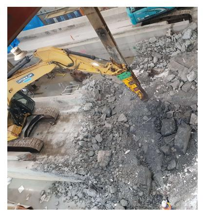
TBM shifting slab breakout
