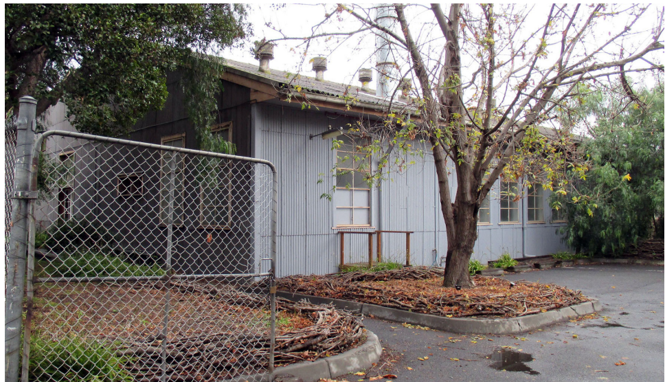
Figure 14-12 Railways Reserve Precinct, 173-199 Laurens Street, North Melbourne (proposed HO1093), the below building is the Former Victorian Railways Carpenters Shop, later Victorian Railways Printing Works (workshop 1), viewed from the north-west
