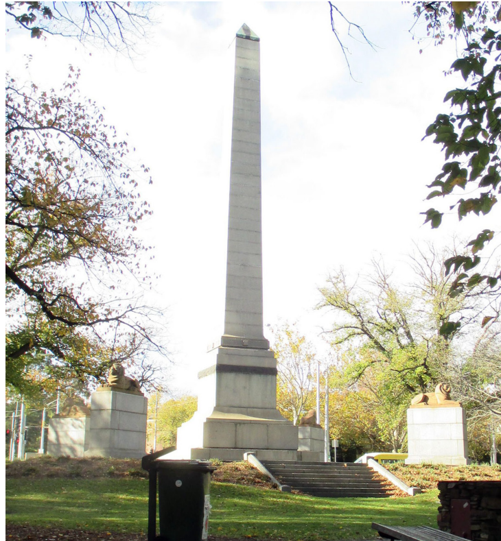
Figure 14-26 The South African Soldiers Memorial viewed from the south (from Albert Road)
