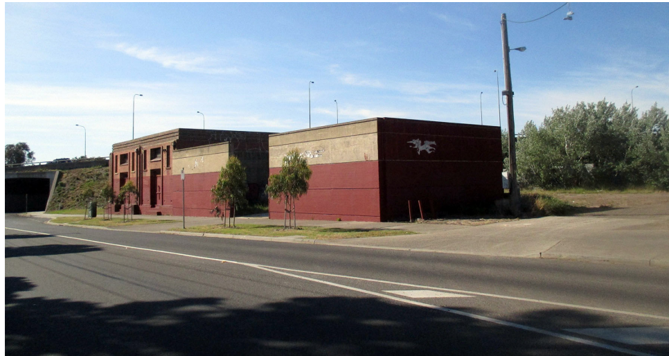
Figure 14-30 Cross Street Electrical Substation (HO192) viewed from the north-west: the brick substation is at left with the concrete walls to the switching yard at right
