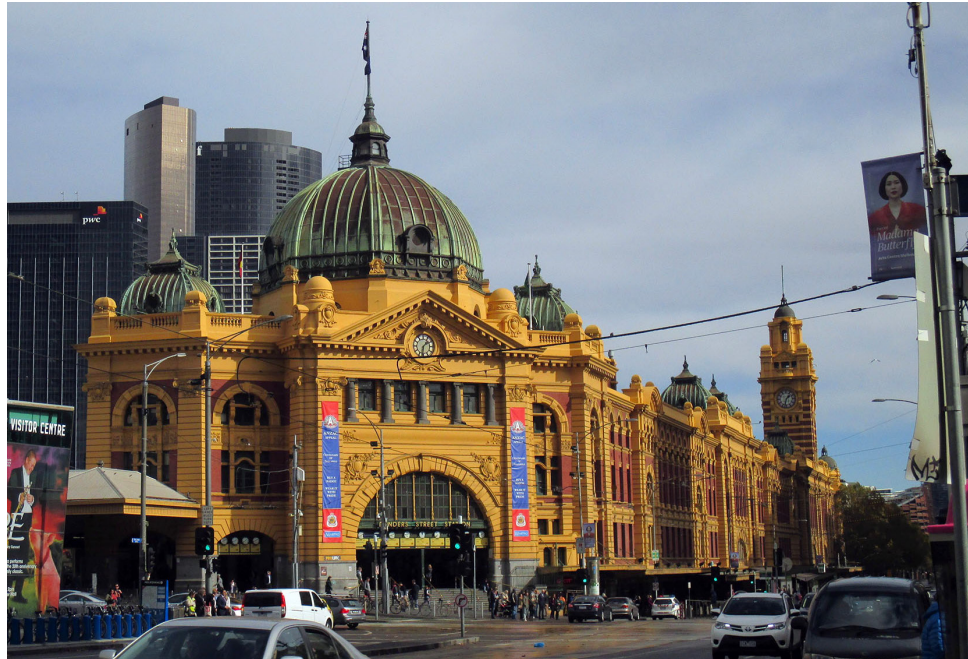
Figure 14-21 Young and Flinders Street Railway Station (VHR H1083) viewed from the north-east
