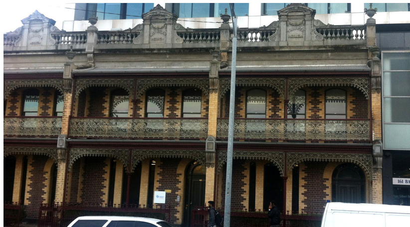
Figure 14-15 Terrace houses in Barry Street, Carlton, Carlton Precinct HO1
