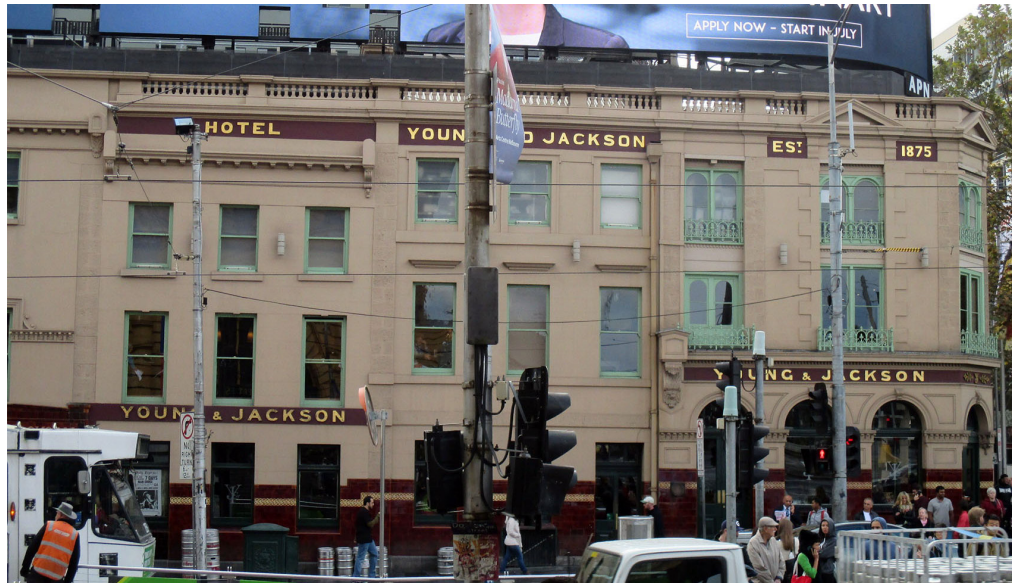
Figure 14-20 Young and Jackson's Princes Bridge Hotel (VHR H0708) Swanston and Flinders streets as viewed from the south
