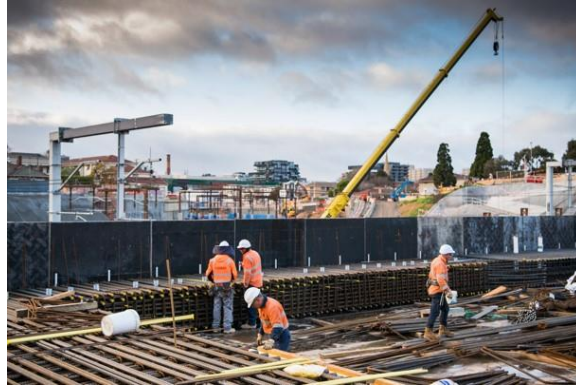
Form work and reinforcement
