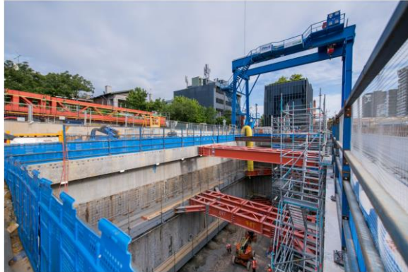
Gantry crane and strutting
