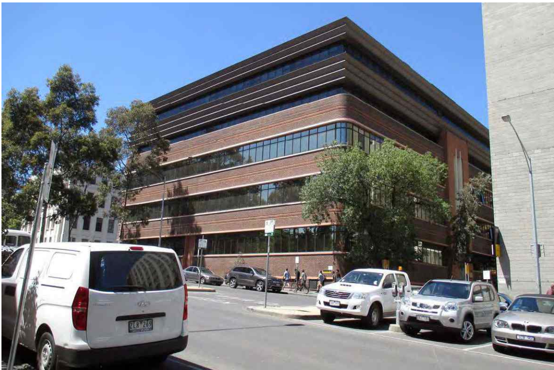
Figure 105 RMIT Building 9, (VHR H1506) viewed from the north; to the south side of Franklin Street
