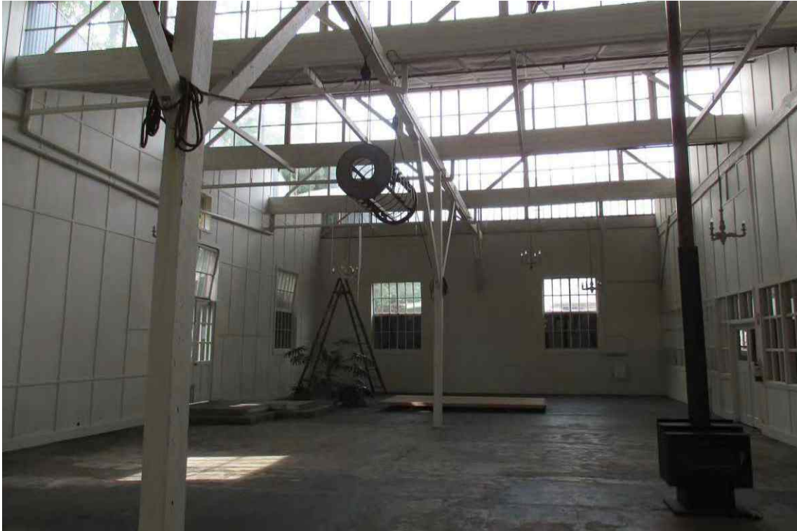
Figure 73 Interior of the Former Victorian Railways Carpenters Shop at the Railways Reserve Precinct, 173-199 Laurens Street, North Melbourne (proposed HO1093)
