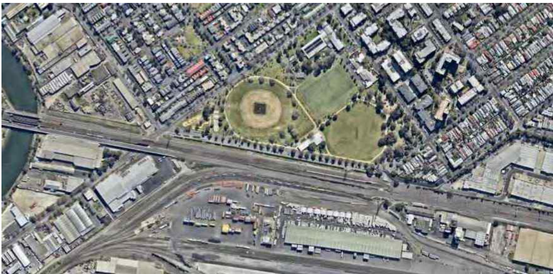
Figure 12 September 2015 aerial image of the western portal precinct and JJ Holland Park Source: Nearmap
