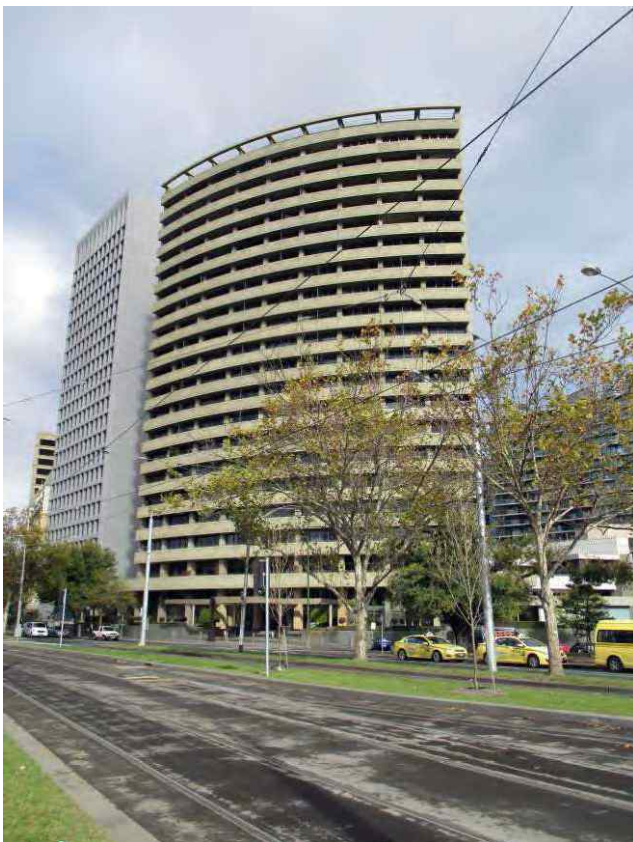
Figure 167 Former BP House (H0319) 1-29 Albert Road, viewed from the north
