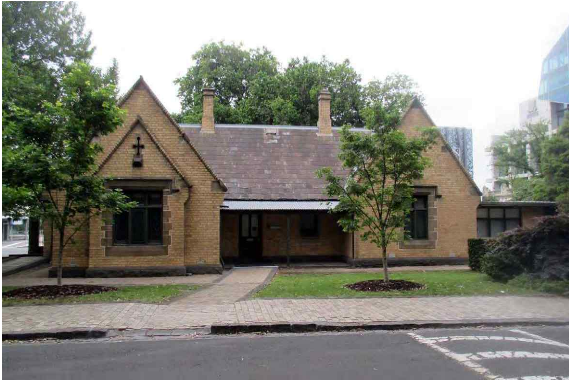
Figure 86 Gatekeeper's Cottage, University of Melbourne (VHR H0919); viewed from the north; note the modern single-storey addition to the west side of the Cottage
