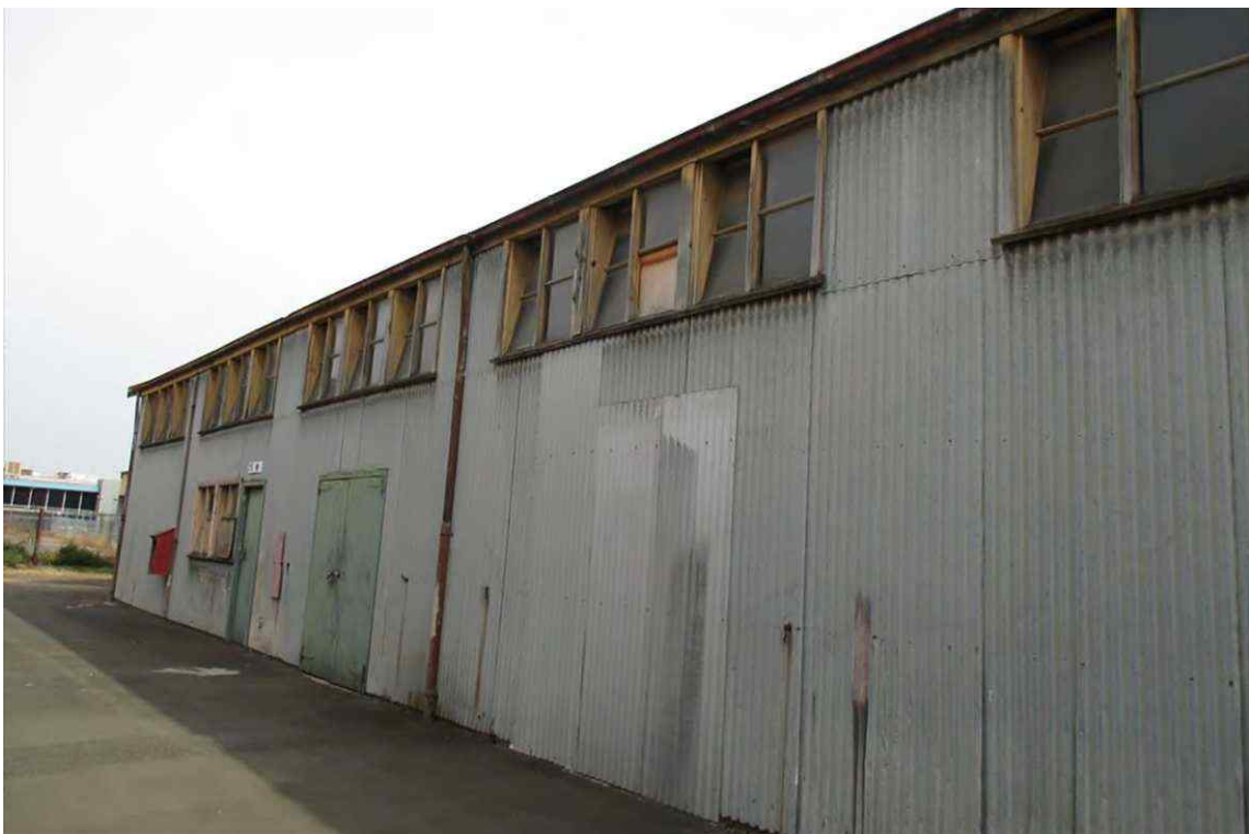
Figure 76 Exterior of the northern workshop at the Railways Reserve Precinct, 173-199 Laurens Street, North Melbourne (proposed HO1093)
