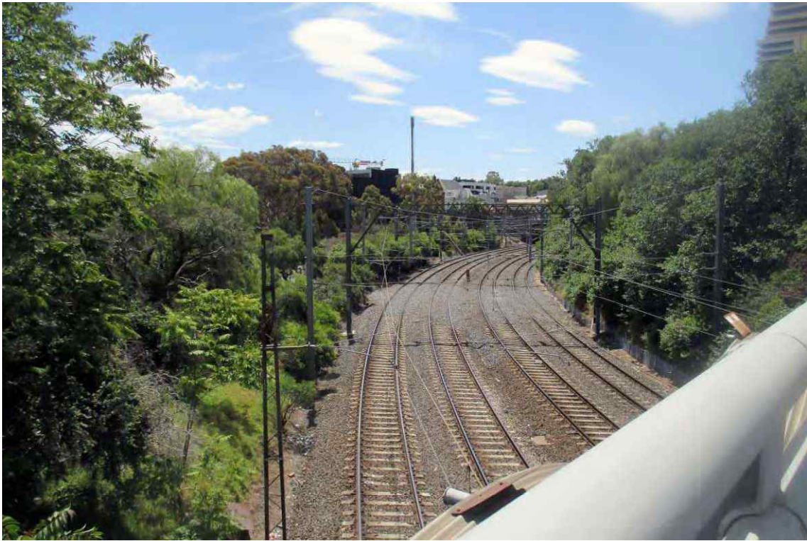
Figure 197 Rail cutting west of the William Street bridge, view looking to the north-east
