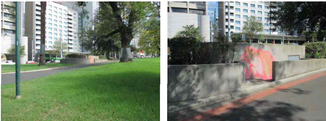
Figure 212 Vent structure on the eastern edge of the Treasury Gardens
