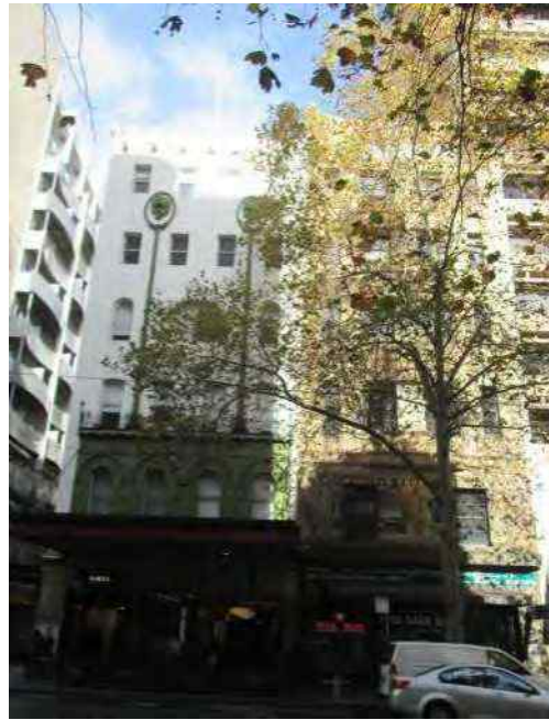
Figure 119 Former Fourth Victoria Building (VHR H1542) at left, with the facade to Newspaper House with the Napier Waller Mosaic (VHR H0447) to the right
