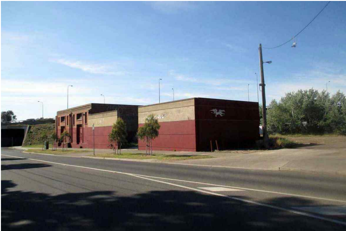
Figure 206 Cross Street Electrical Substation (HO192) viewed from the north-west: the brick substation is at left with the concrete walls to the switching yard at right
