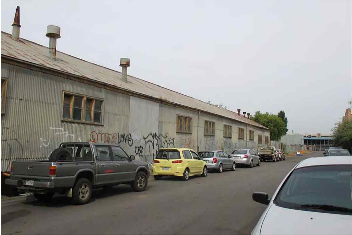
Figure 77 Northern elevation of the northern workshop at the Railways Reserve Precinct, 173-199 Laurens Street, North Melbourne (proposed HO1093)
