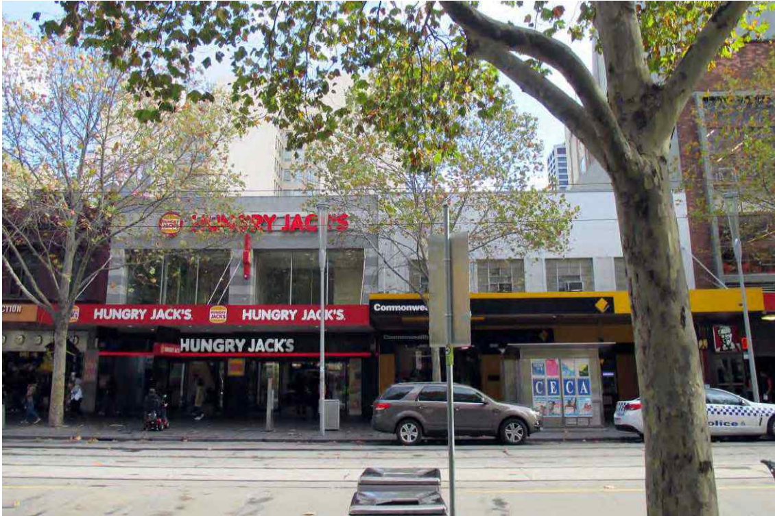
Figure 146 Ungraded building at 15-25 Swanston Street
