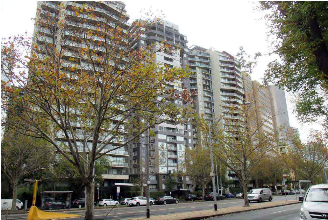
Figure 164 Large towers on the south side of St Kilda Road
