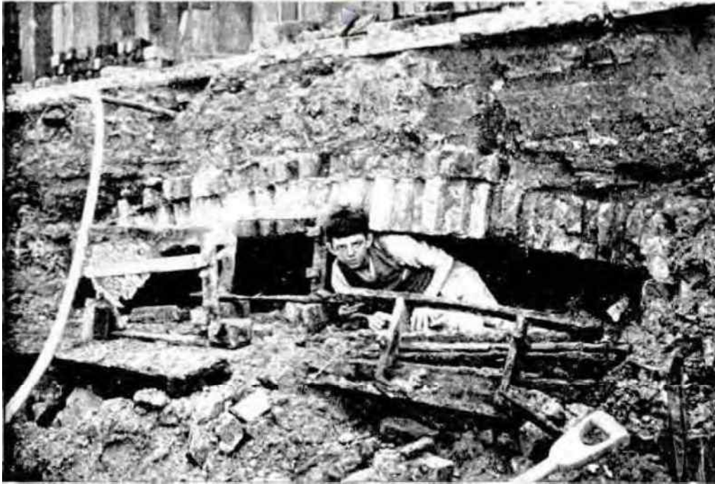
Figure 27 Brick oven located during construction works, 1904 Source: Leader , 16 April 1904, p. 33
