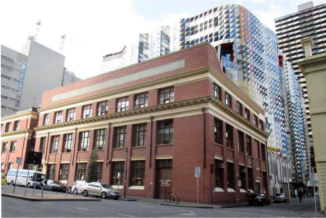
Figure 108 67-77 Franklin Street, Melbourne (part HO1042) viewed from the west
