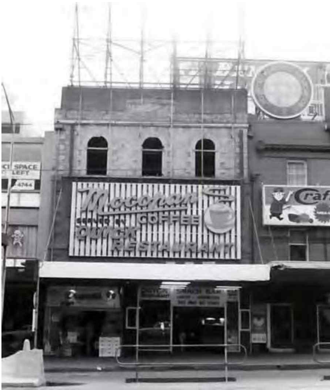
Figure 151 Undated (c. 1978) photograph of 222-224 Flinders Street, with carriageway in use as a shop: Note bricked over parapet and signage to facade. Source: National Trust of Australia (Victoria), via http://vhd.heritage.vic.gov.au/search/nattrust_result_detail/64969
