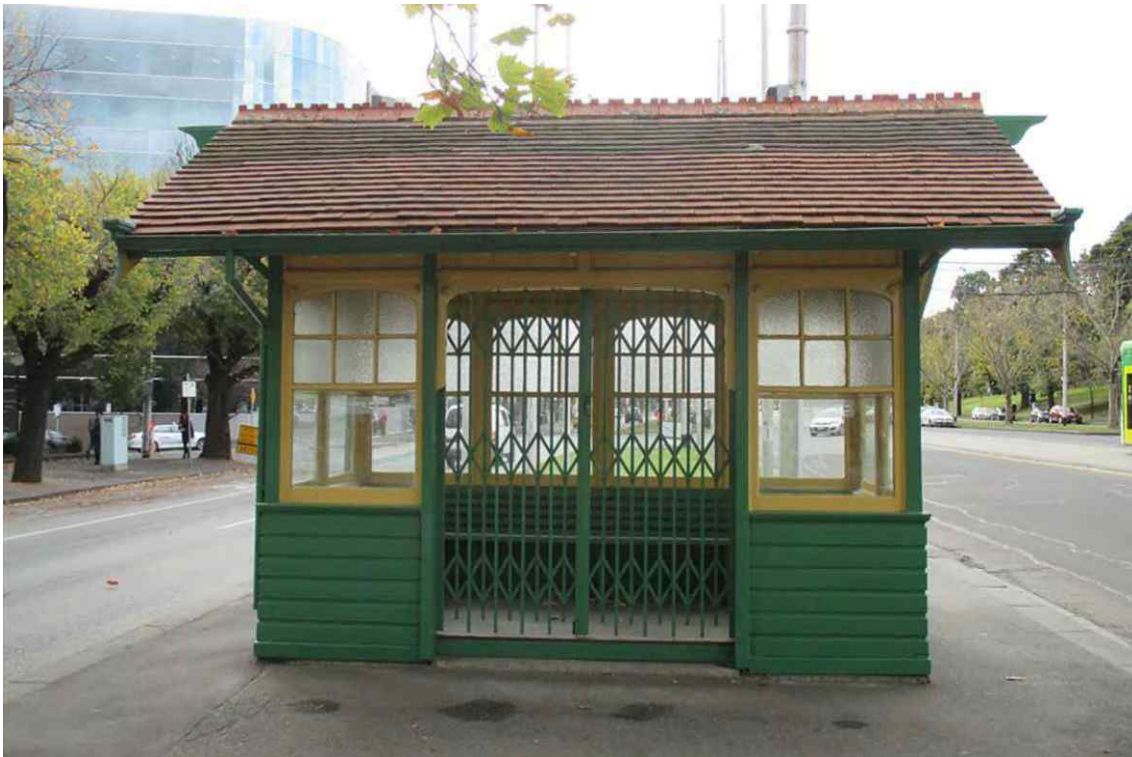
Figure 185 View of the Tram Shelter looking north along St Kilda Road
