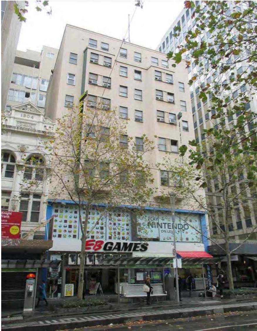
Figure 137 Former Graham Hotel, 67-73 Swanston Street
