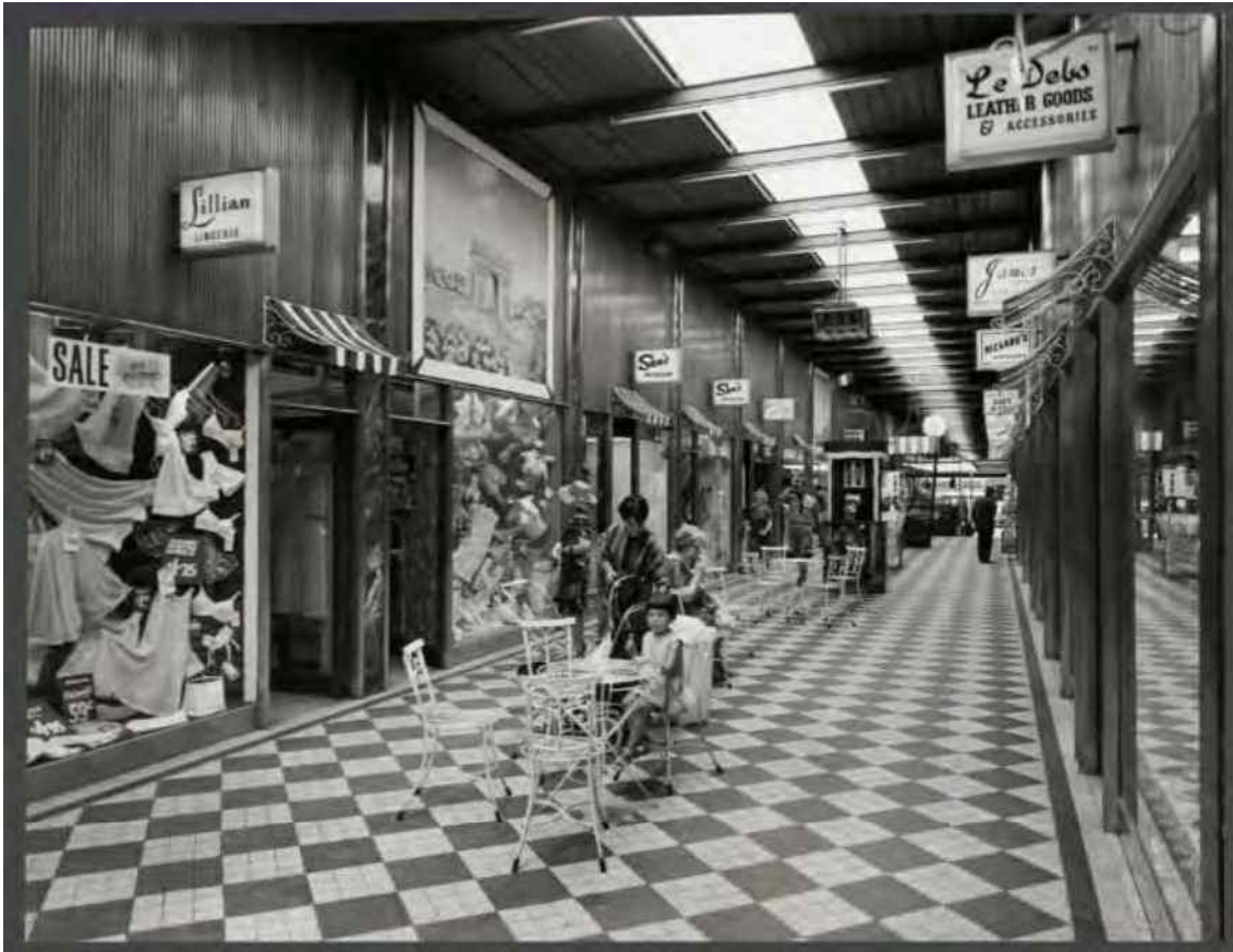
Figure 143 Interior of the arcade looking towards Flinders Street, c. 1969 Source: Wolfgang Sievers collection, State Library of Victoria
