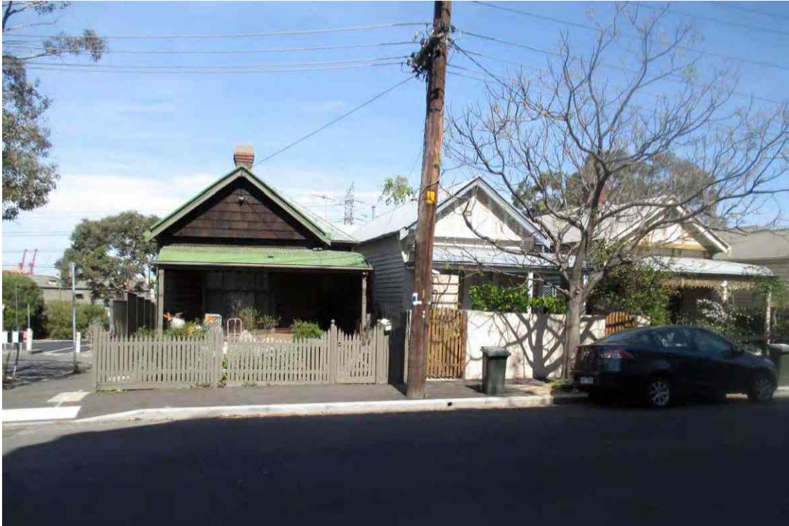
Figure 53 From left; Nos 1, 3 and 5 Altona Street, Kensington within HO9 Kensington Precinct (all D grade, Level 3 streetscape), to be retained
