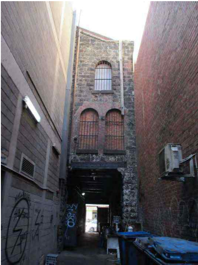
Figure 154 View of the northern elevation of the building (eastern section obscured by later building)
