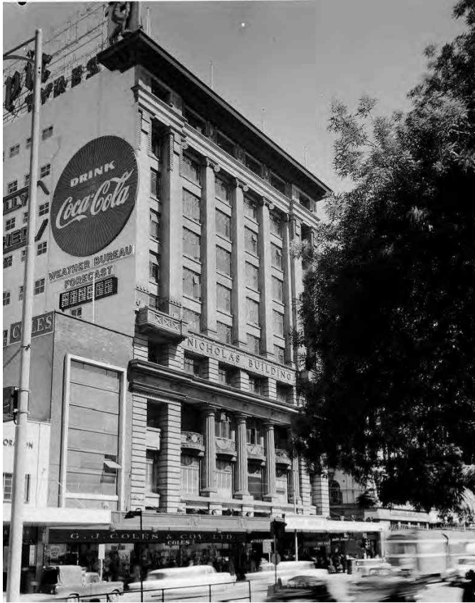
Figure 132 Swanston Street, c. 1962 showing the building at 27-29 Swanston Street, accommodating the GJ Coles store and with continuous canopy from the Nicholas Building Source: State Library of Victoria (photographer Mark Strizic)
