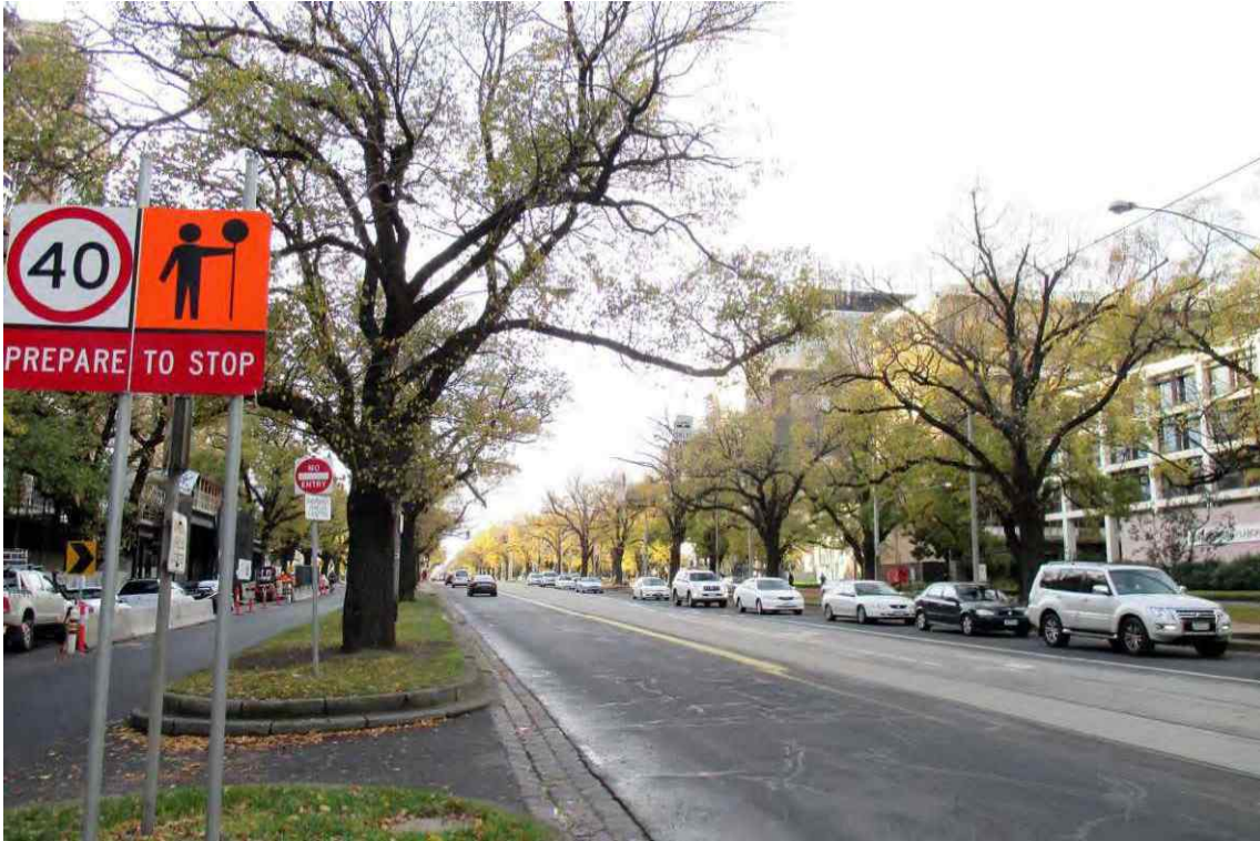
Figure 82 View north along Royal Parade from Grattan Street showing concrete kerbing and bluestone gutters
