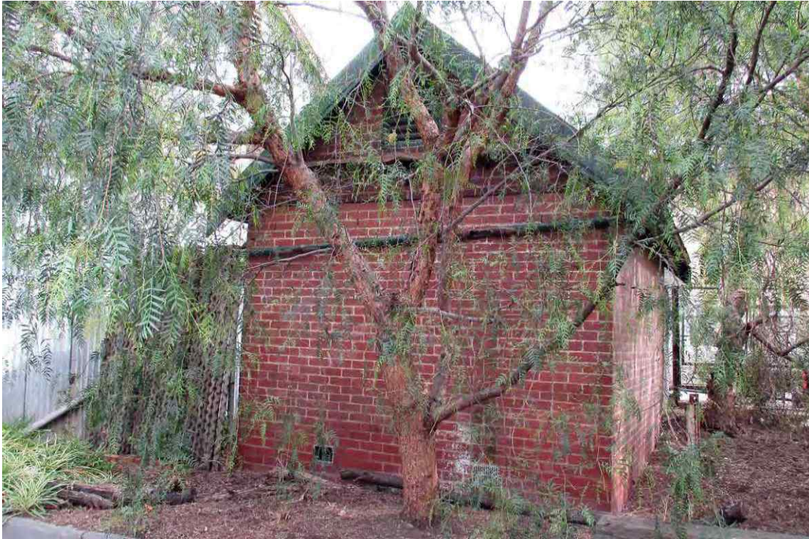
Figure 62 Brick substation within the Railways Reserve Precinct (proposed HO1093) as viewed from the south, within the site
