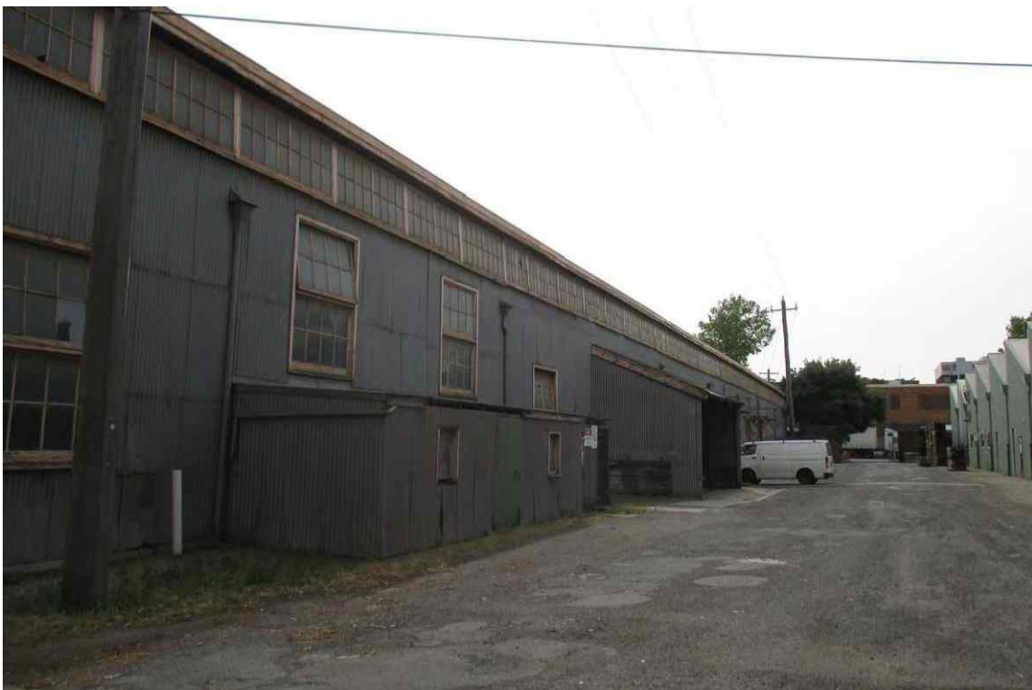
Figure 70 Southern elevation of the Former Victorian Railways Carpenters Shop at Railways Reserve Precinct, 173-199 Laurens Street, North Melbourne (proposed HO1093)
