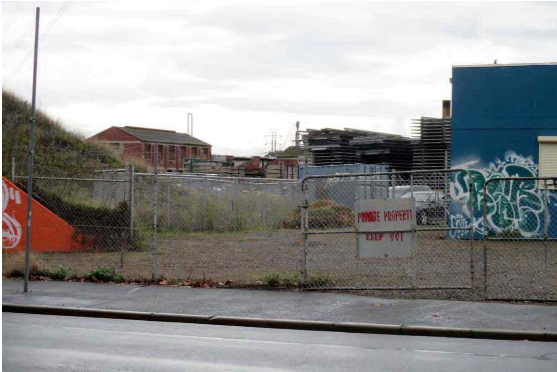
Figure 49 View along the southern boundary of the former Kensington Glue Works site at 1-39 Hobsons Road, Kensington (HO239) as included within the western portal precinct (C grade, Level 3 streetscape), site to be used for construction purposes
