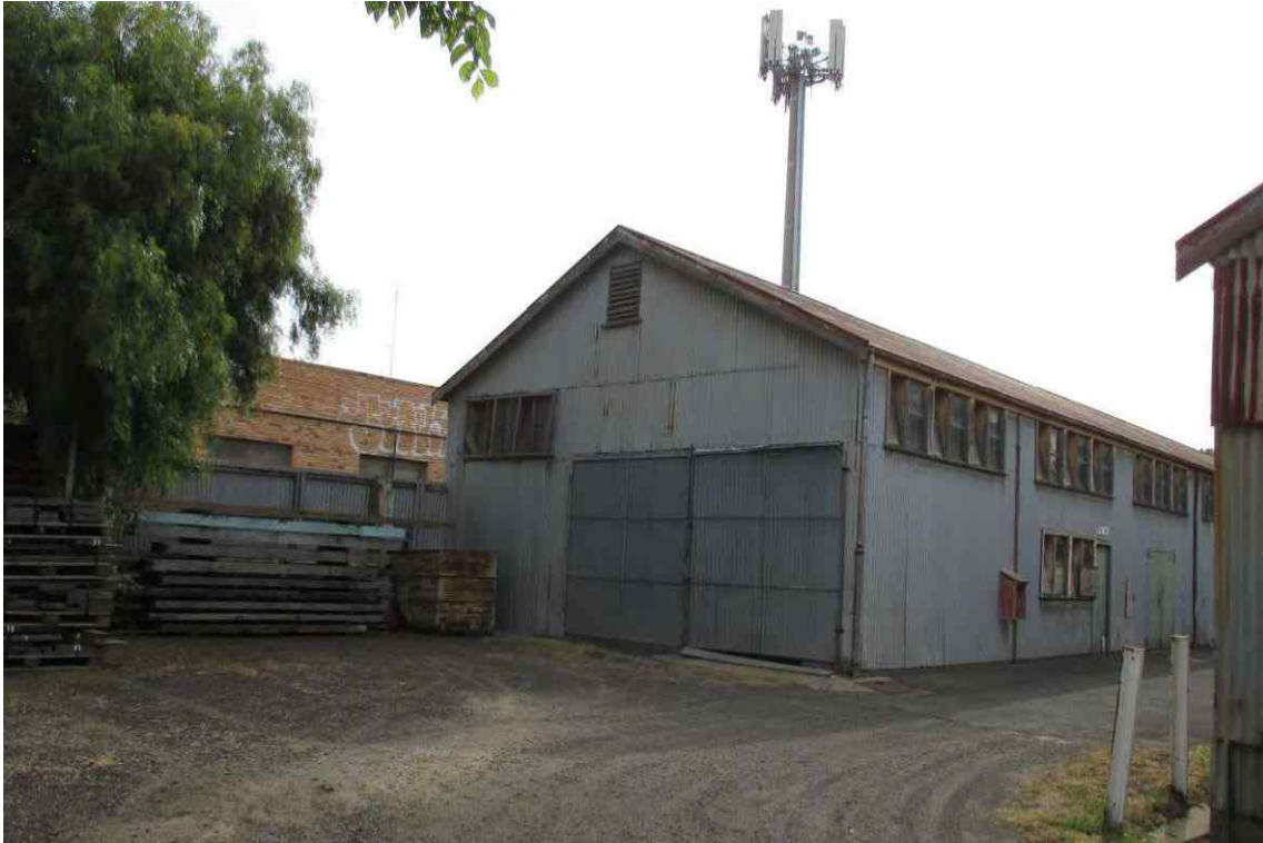
Figure 60 West and south elevation of the northern workshop to Railways Reserve Precinct, 173-199 Laurens Street, North Melbourne (proposed HO1093), with the central shed behind
