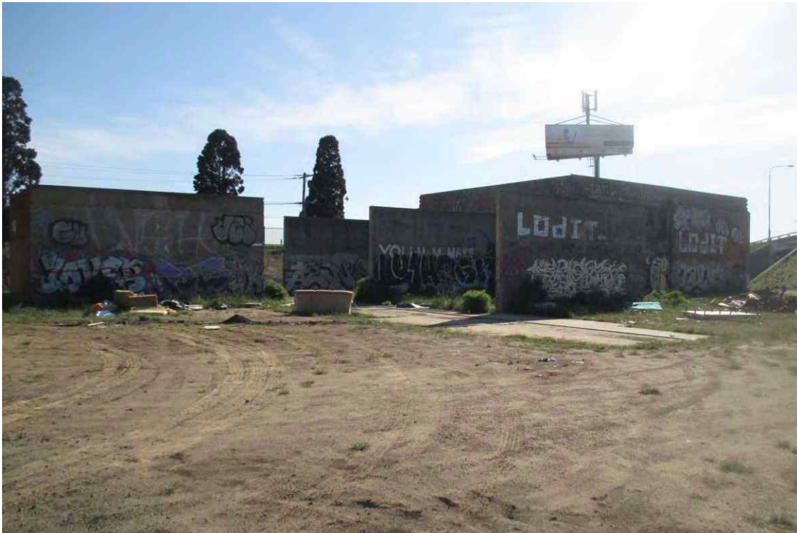
Figure 208 Cross Street Electrical Substation (HO192) viewed from the south-west: note the concrete walls demarcating the former switching yard
