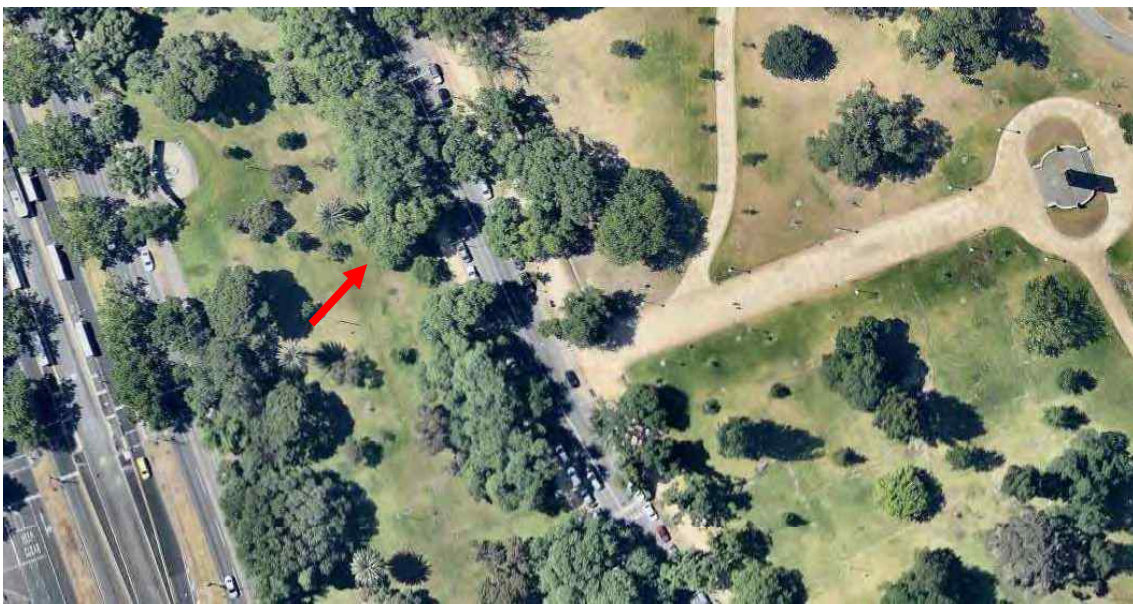
Figure 32 Aerial view showing the context of the proposed emergency shaft location in Tom's Block
