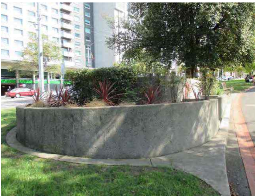
Figure 211 Vent structure within Flagstaff Gardens
