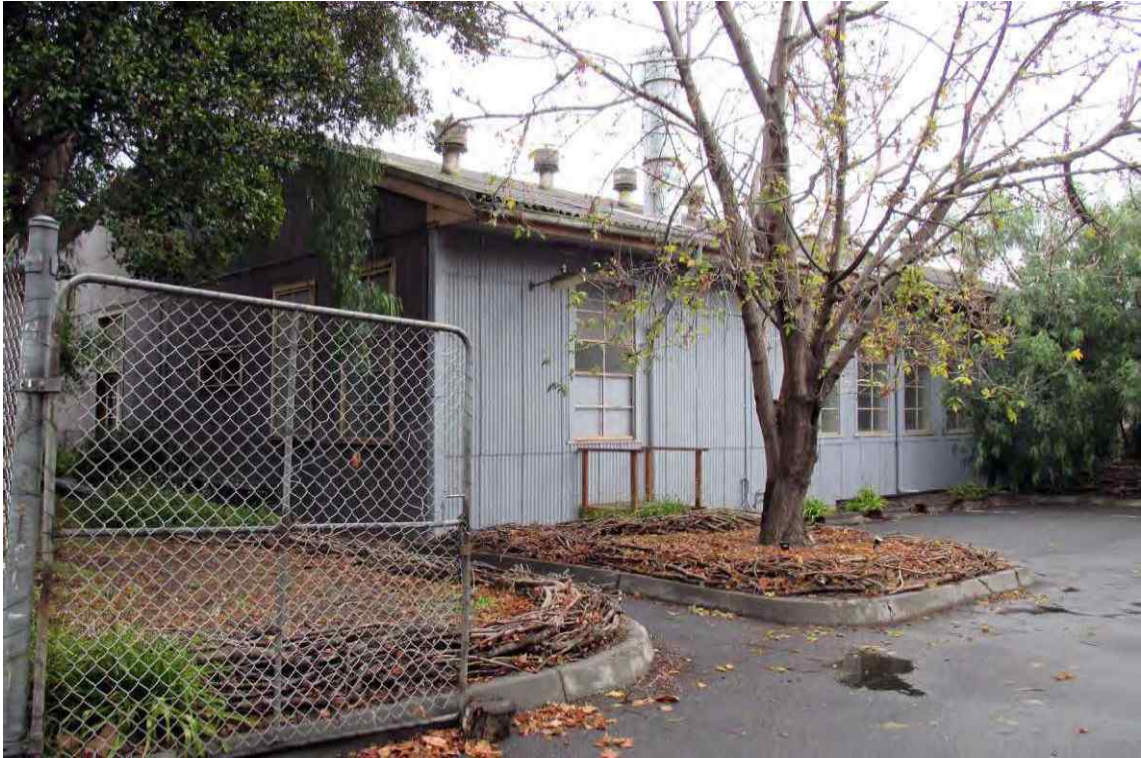
Figure 58 Railways Reserve Precinct, 173-199 Laurens Street, North Melbourne (proposed HO1093), the above building is the Former Victorian Railways Carpenters Shop, later Victorian Railways Printing Works (workshop 1), viewed from the north-west
