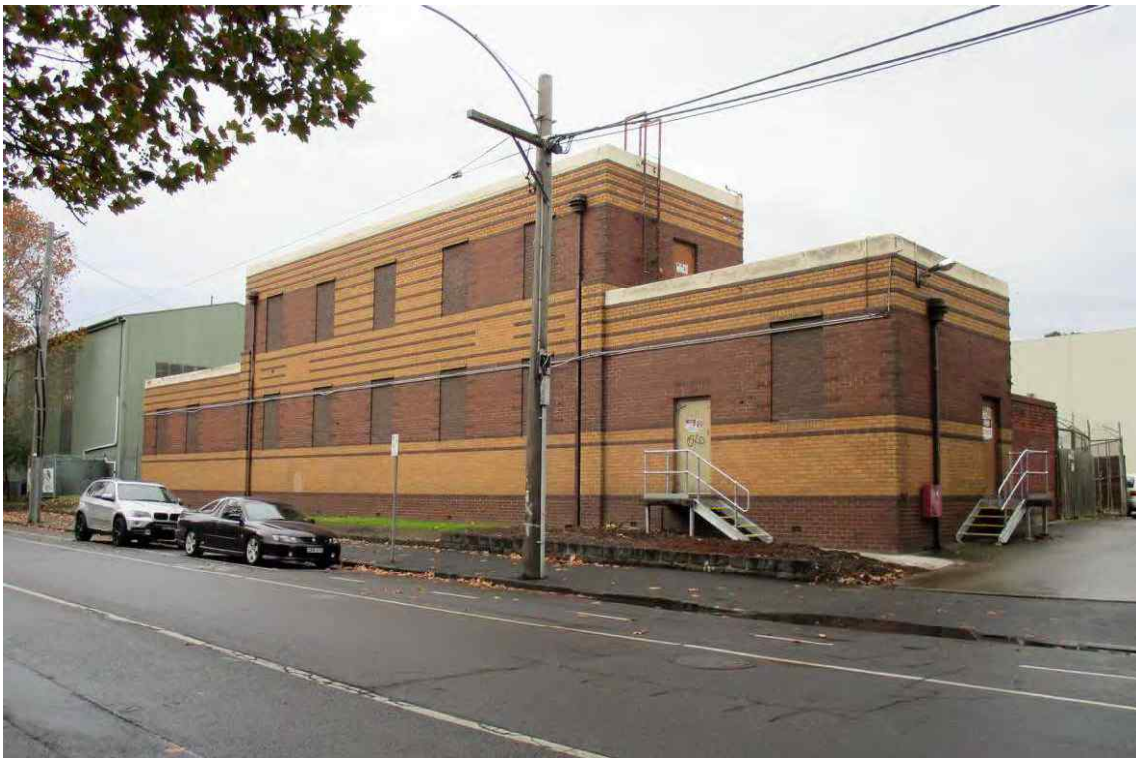
Figure 63 Melbourne City Council Electric Supply substation and coal yard later Citipower, 146-166 Laurs Street, North Melbourne (proposed HO1111)
