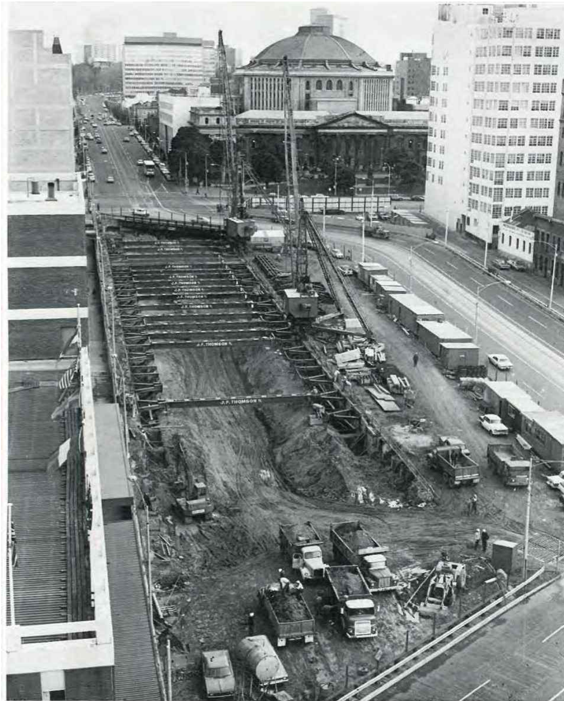
Excavation for Museum station under-street structure followed the placing of soldier piles around the perimeter. Earlier contracts provided for demolition of buildings and diversion of roadway and services.
