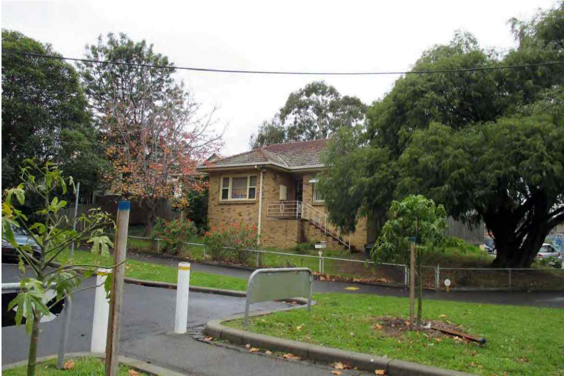
Figure 55 135-141 Ormond Street, Kensington viewed from the south-west (proposed to be demolished in the Concept Design)
