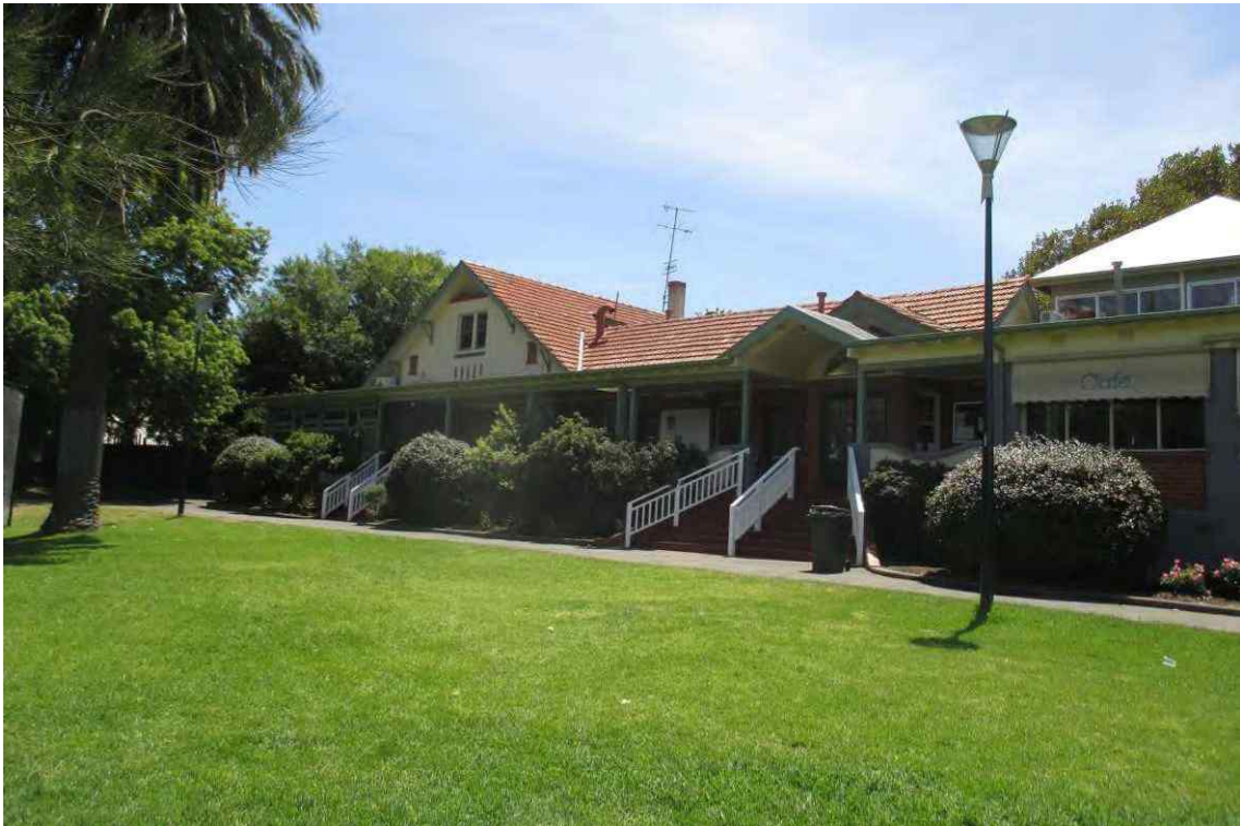
Figure 15 View of open space to the west of the Tennis Club and Community Centre
