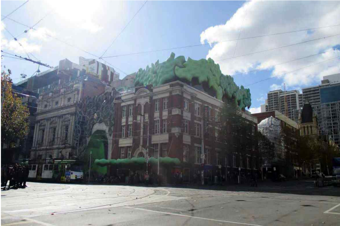
Figure 113 Building 22, 330-334 Swanston Street, Melbourne (C grade, Level 2 streetscape, at centre); RMIT Storey Hall (VHR H1498, with later addition at left); Former Foresters Hall (VHR H1495, under scaffold at right) viewed from the south
