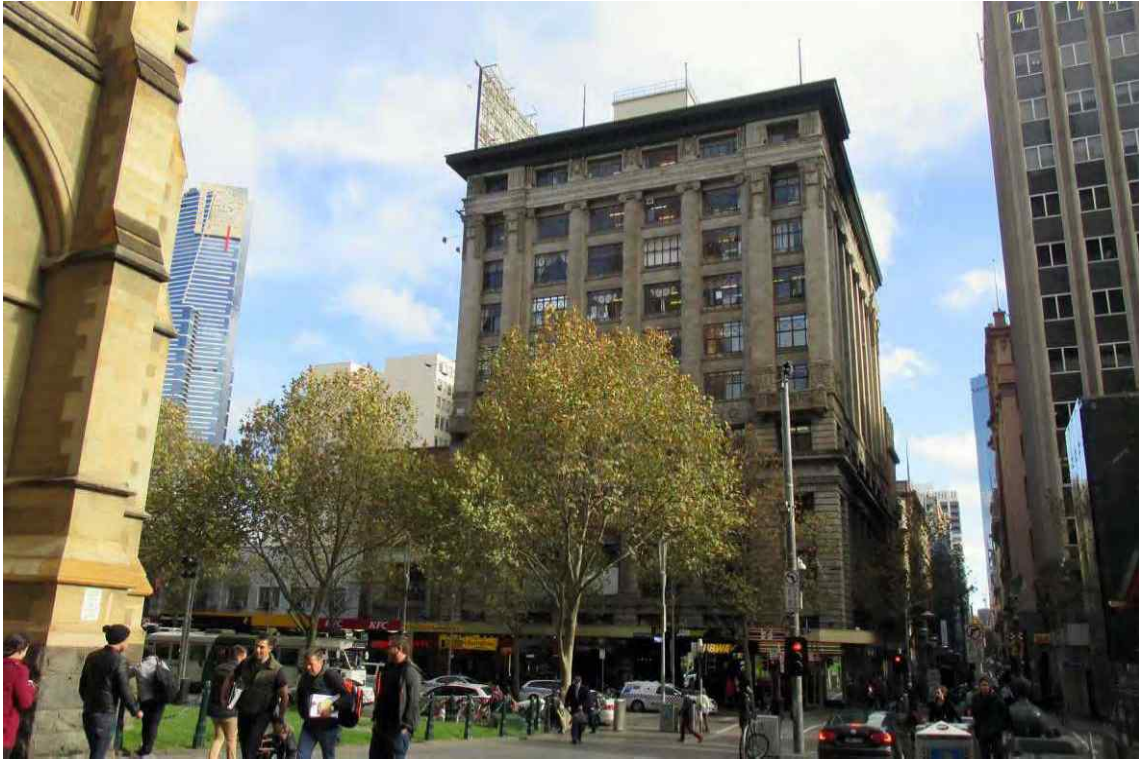
Figure 123 Nicholas Building (VHR H2119), 31-41 Swanston Street viewed from the east
