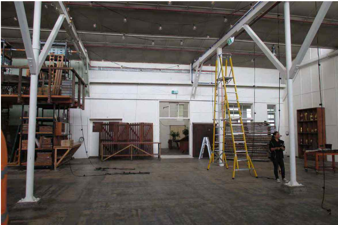
Figure 74 Interior of the Former Victorian Railways Carpenters Shop at the Railways Reserve Precinct, 173-199 Laurens Street, North Melbourne (proposed HO1093) looking north
