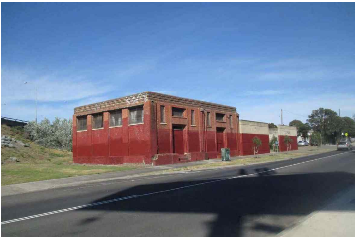
Figure 207 Cross Street Electrical Substation (HO192) viewed from the north-east
