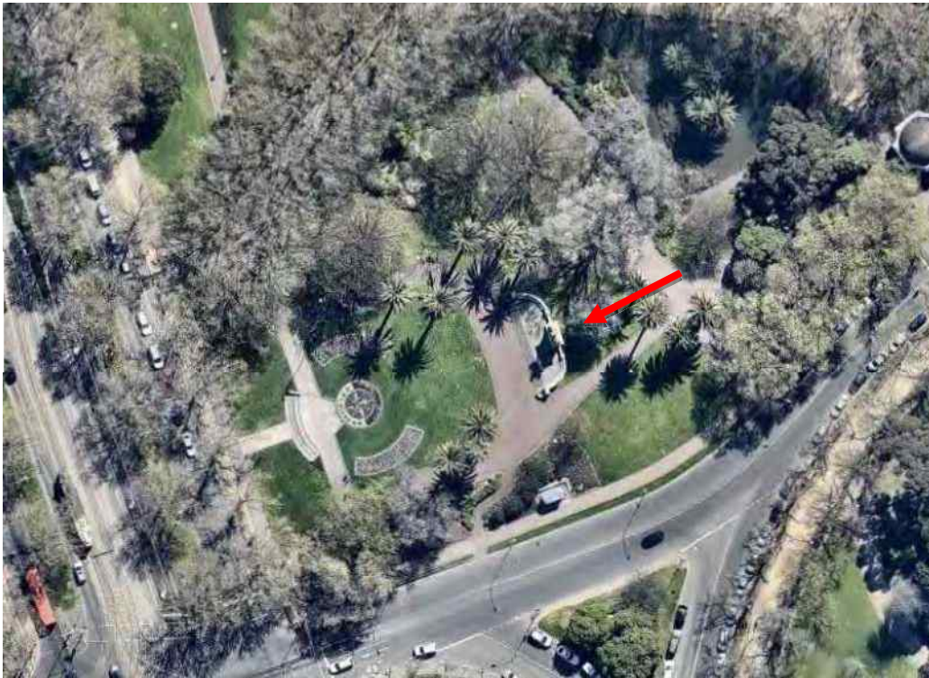
Figure 22 Aerial view of the location of the proposed emergency access shaft at Linlithgow Avenue with the King Edward VII Memorial (red arrow), the Floral Clock and palms: refer to Figure 30 for the location of the emergency access shaft Source: Nearmap, 13 September 2015
