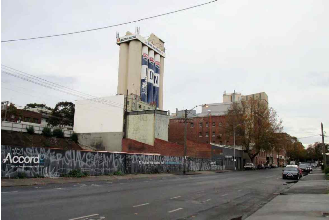
Figure 64 Thomas Brunton & Co flour mill complex, later Weston Milling factory, 24-78 Laurens Street (proposed for inclusion in HO455)
