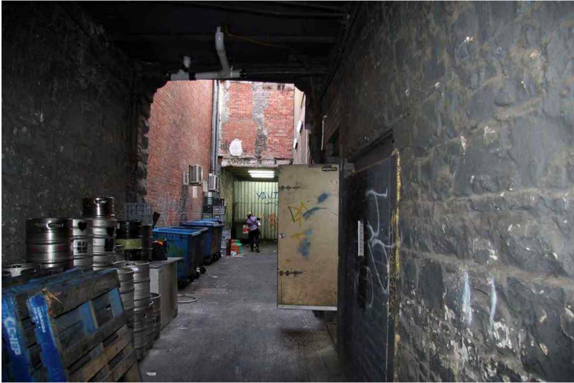
Figure 153 View north from within the carriageway
