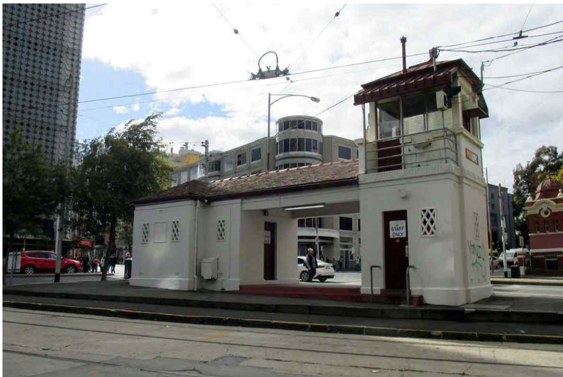
Figure 103 Tramway Signal Cabin, Waiting Shelter and Conveniences, (VHR H1686) within the roadway at the intersection of Swanston and Victoria streets
