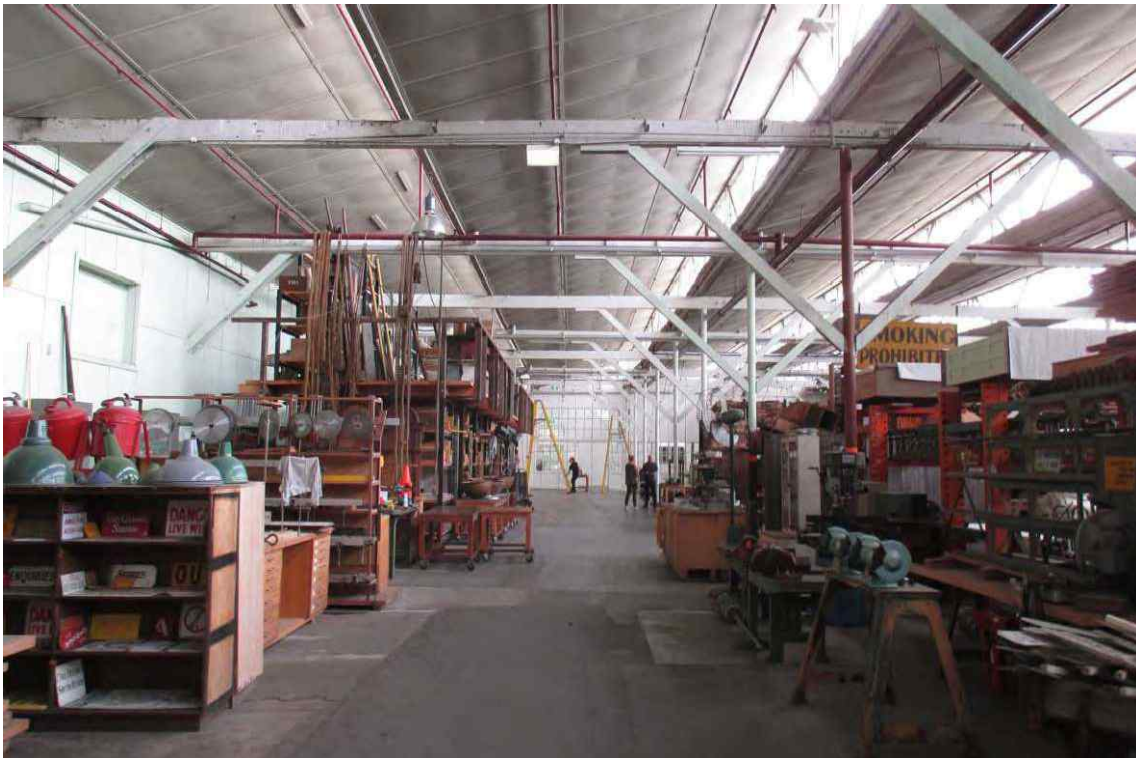
Figure 72 Internal view of the Former Victorian Railways Carpenters Shop at the Railways Reserve Precinct, 173-199 Laurens Street, North Melbourne (proposed HO1093) looking north
