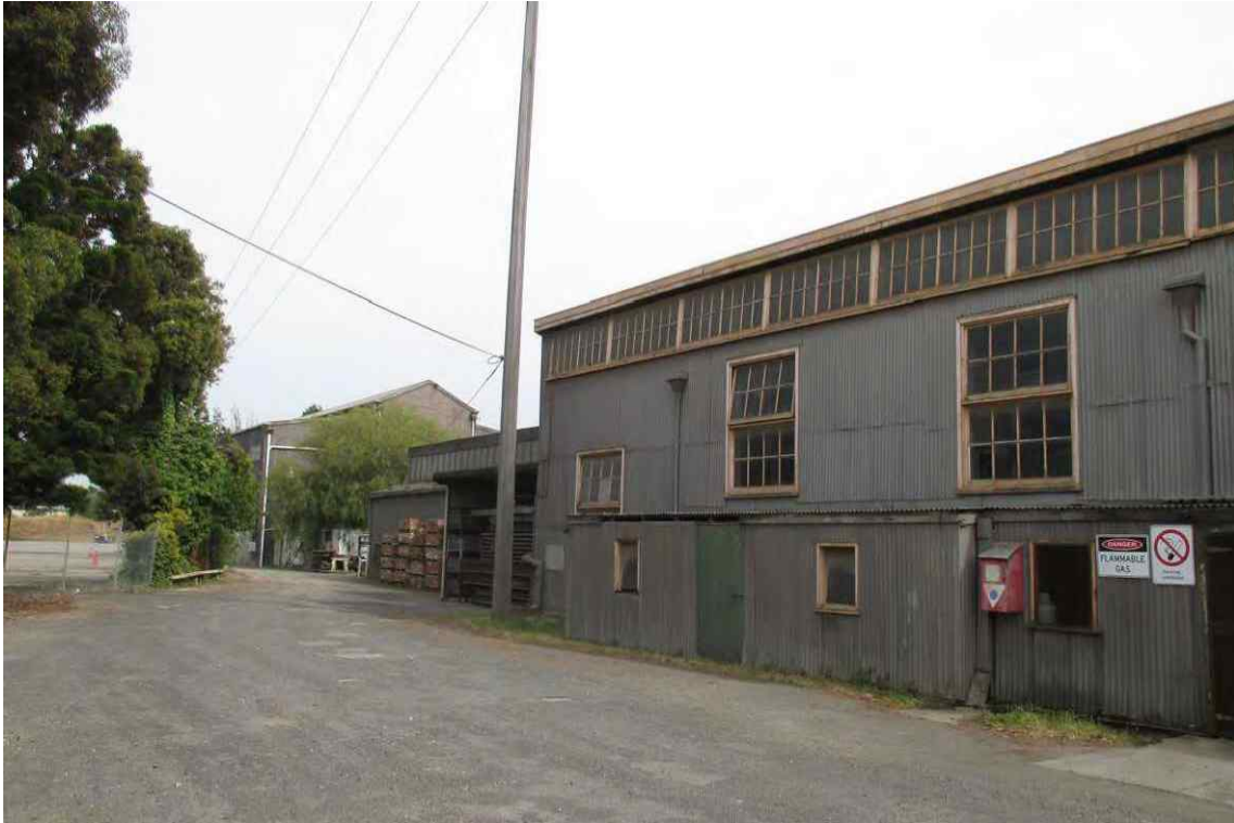
Figure 71 Southern elevation (looking west) of the Former Victorian Railways Carpenters Shop at the Railways Reserve Precinct, 173-199 Laurens Street, North Melbourne (proposed HO1093)
