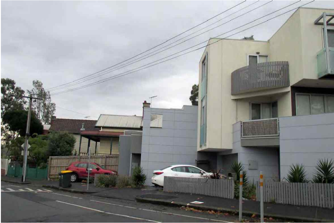
Figure 51 Townhouse development at 9 and 13 Childers Street, Kensington at the corner of Childers and Tennyson streets viewed from the east (proposed to be demolished as part of the Concept Design)
