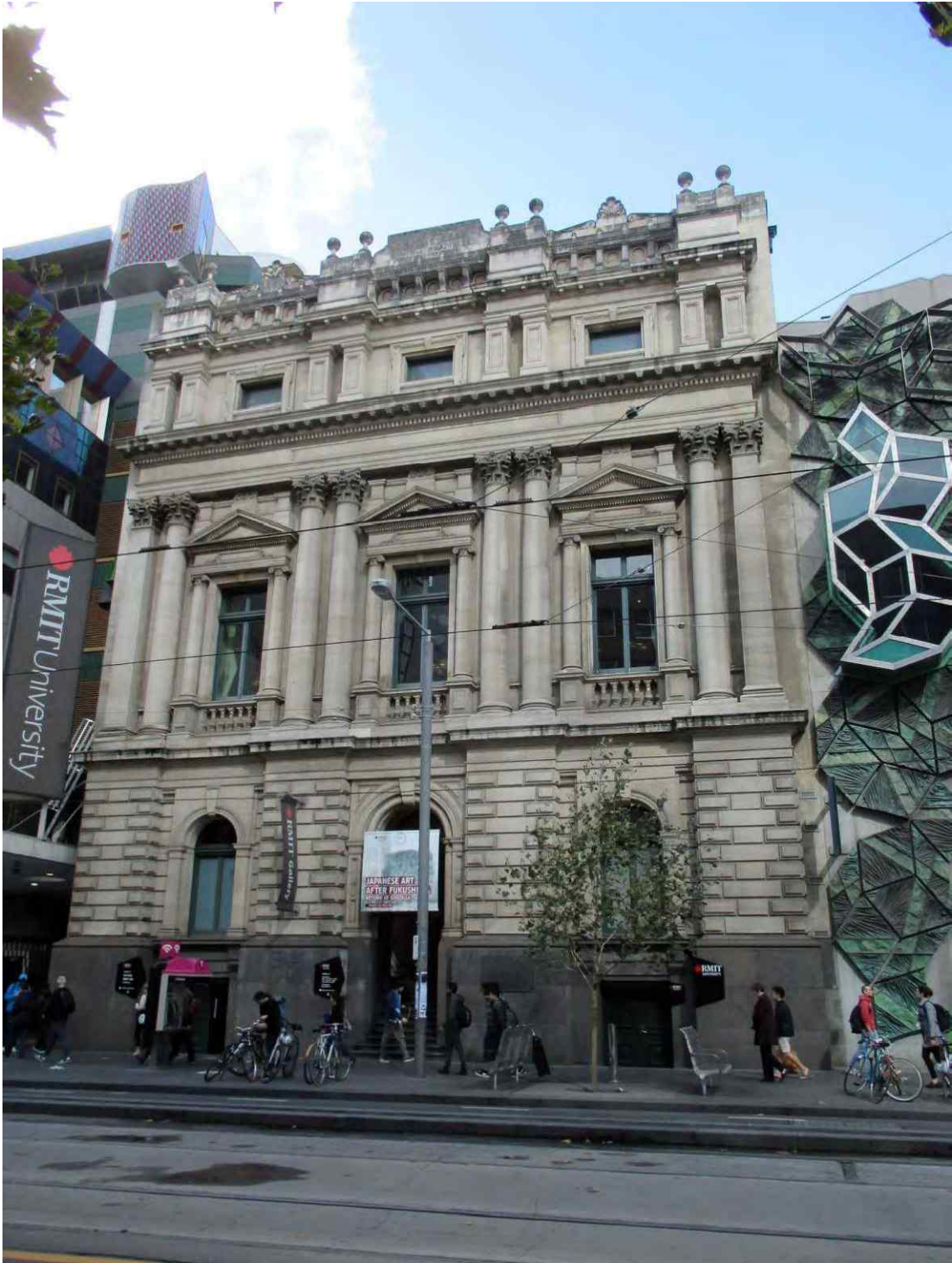
Figure 106 Storey Hall, 344-346 Swanston Street (VHR H1498) on the east side
