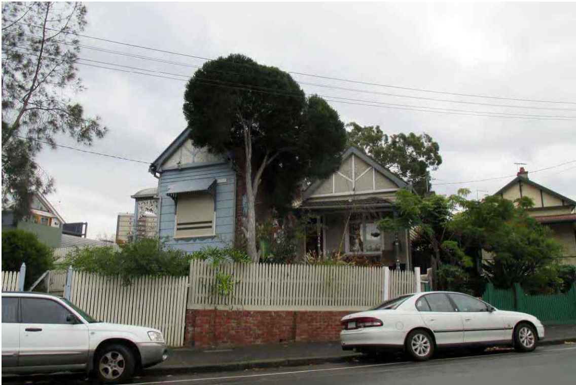
Figure 50 Edwardian period residences within HO9 Kensington Precinct at Nos 1 to 5 Childers Street, Kensington (all D grade, Level 3 streetscape) viewed from the south (proposed to be demolished as part of the Concept Design)
