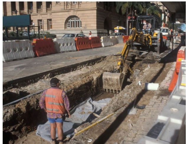
Figure 1. Installation of street tree pits
