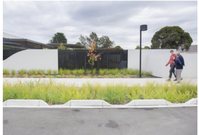
Figure 3: Example of a passively irrigated garden bed with surface inlets (source: City of Darebin)
