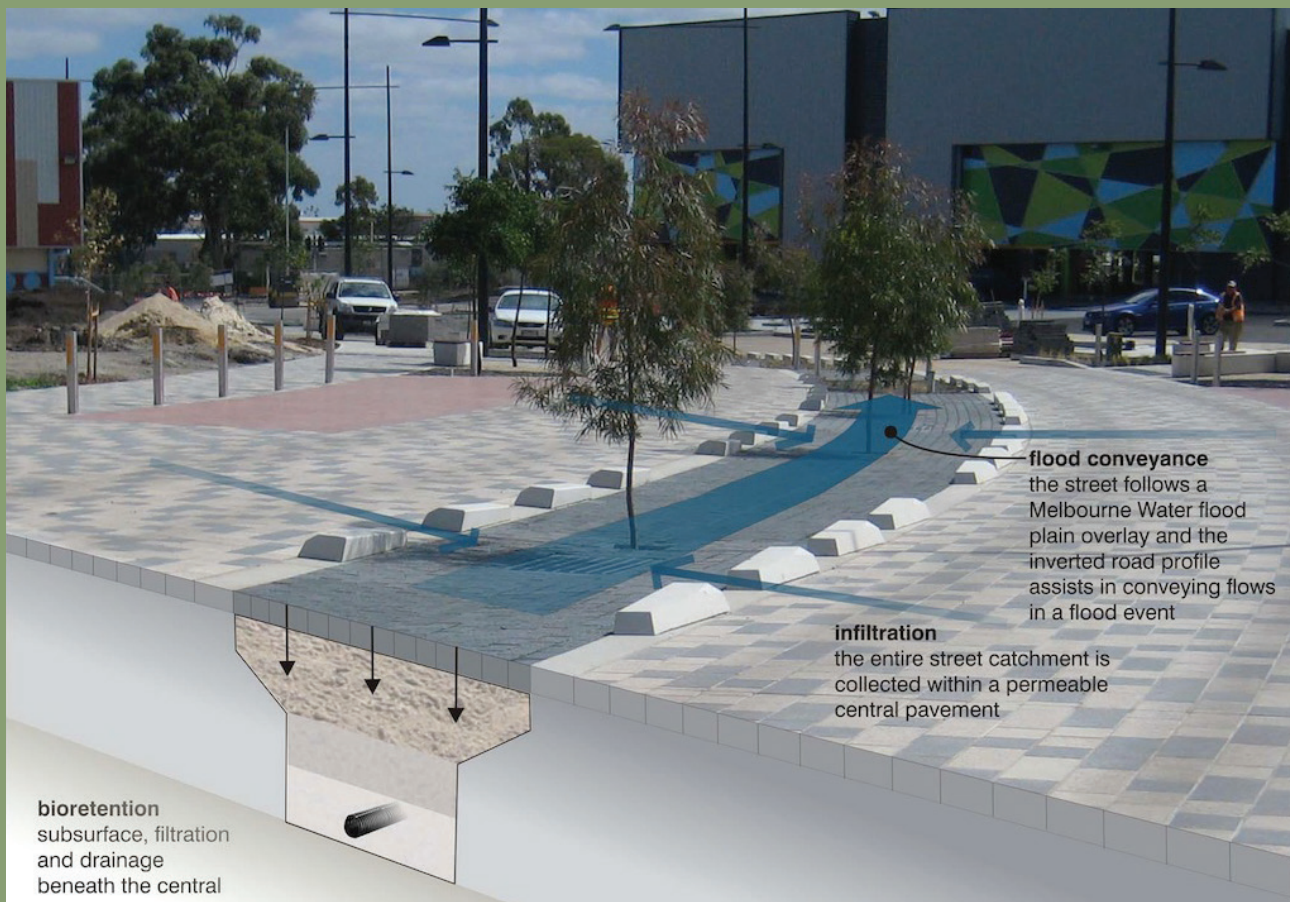
Figure 3: The Tanderrum Way, Broadmeadows. Image: Hydroston.com.au
