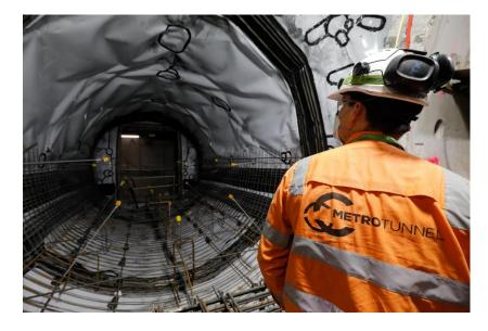
Steelfixing installed before concrete linings can be poured
