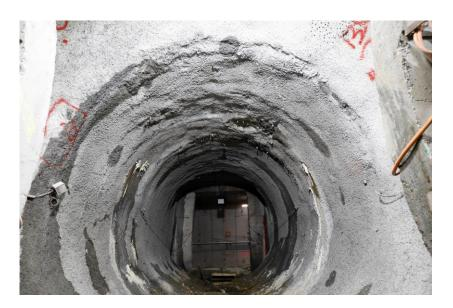
Cross passage shotcreted before permanent lining works completed
