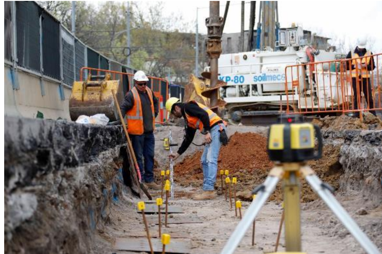
(Retaining Wall: Southern Box)
