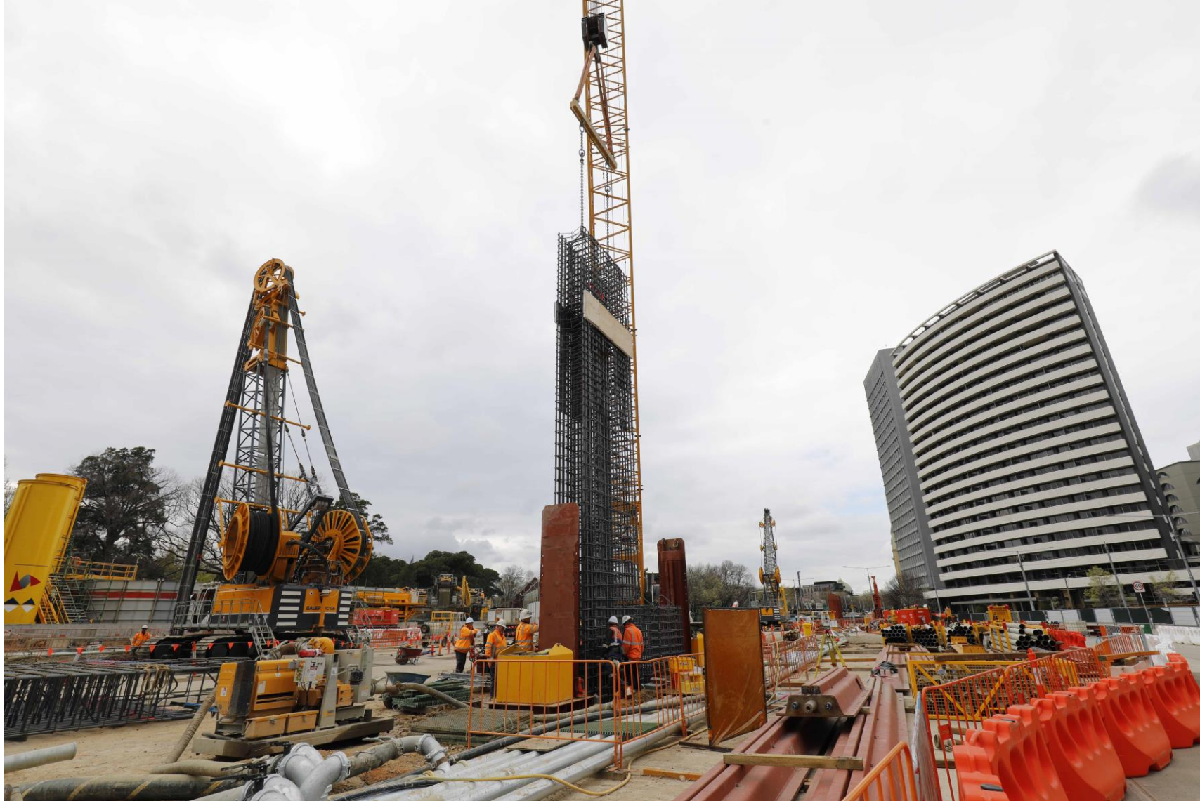
(D-wall cage being lowered into place)
