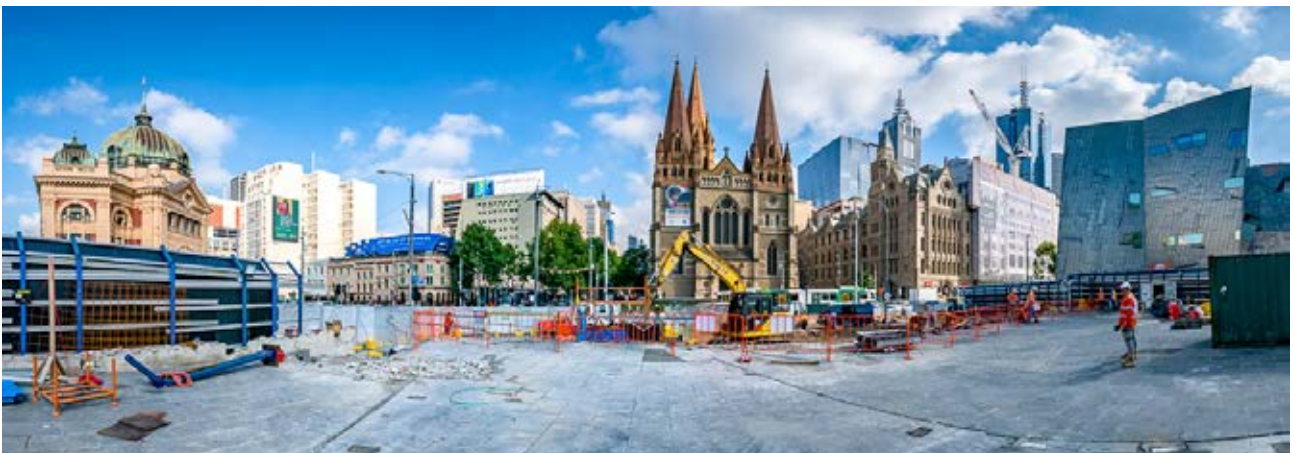
Federation Square site
