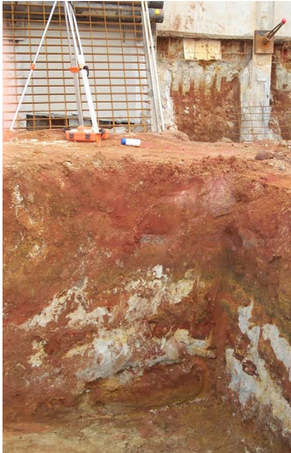
Plate 11: Brighton Group materials exposed in a basement excavation
