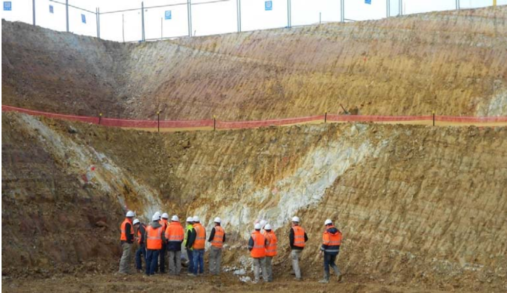
Plate 6: Weathered dyke exposed in open excavation within Melbourne Formation (Golder archives)
