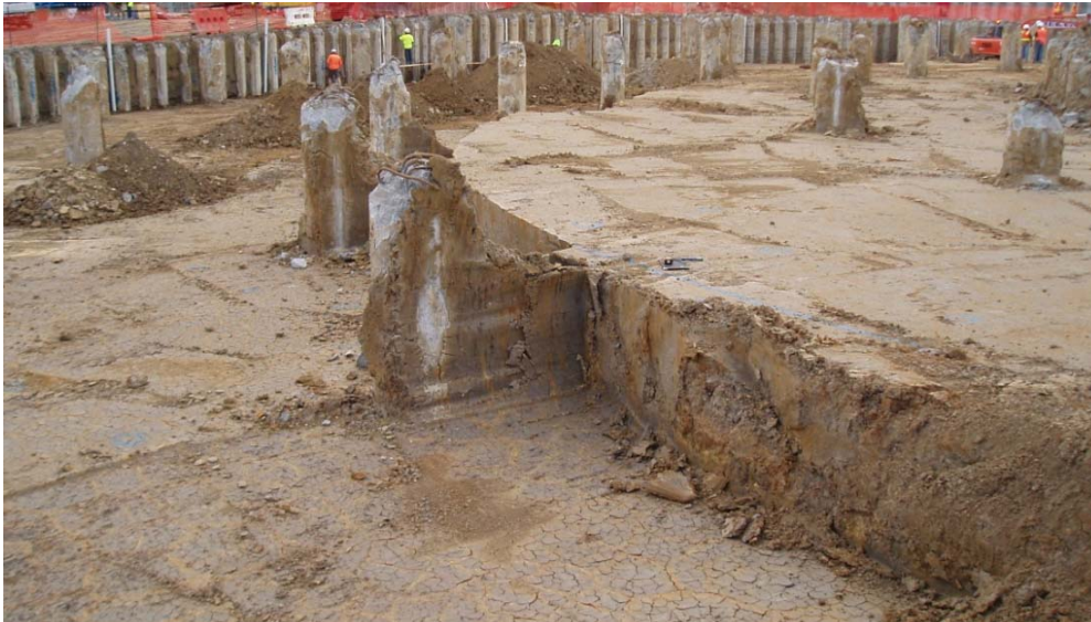
Plate 14: Base of Excavation within Fishermens Bend Silt, Southbank
