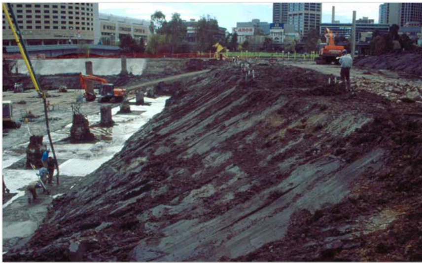
Plate 16: Coode Island Silt Exposed in Excavation, Southbank (Golder archives)
