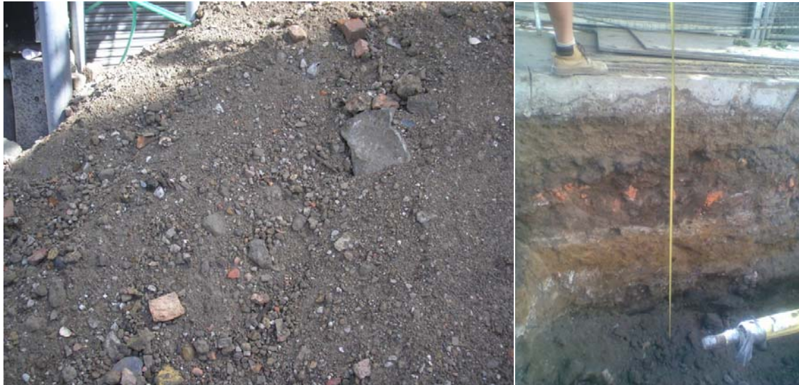
Plate 17: Examples of Fill material encountered in excavations in Southbank (Golder archives)
