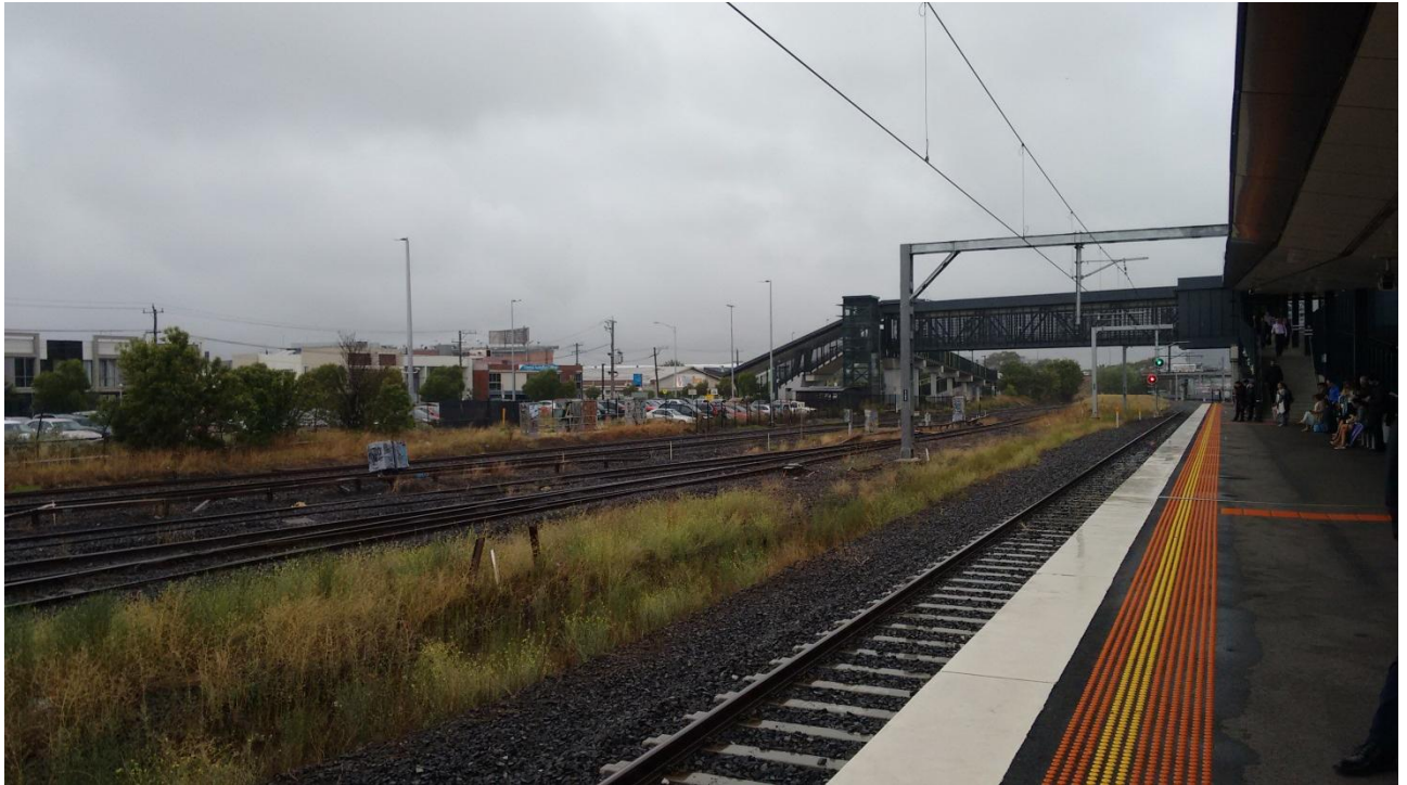
Figure 14-1 Location of the new train platform looking east
