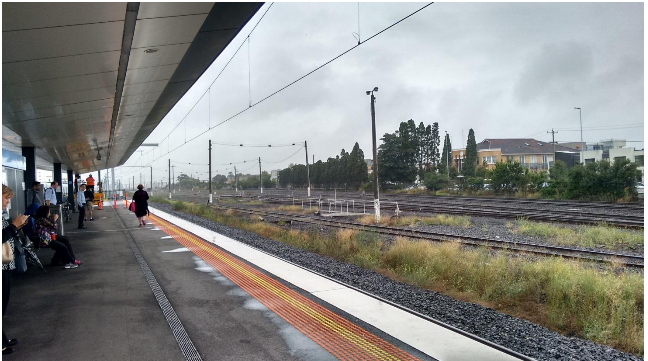
Figure 14-2 Location of the new platform looking west
