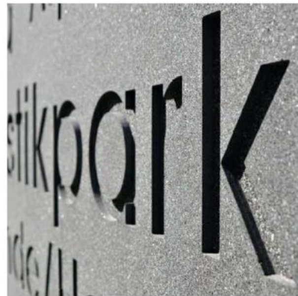
CUSTOM CONCRETE FORM LINER WITH 50MM PATTERN DEPTH. FINAL PATTERN TBC.
