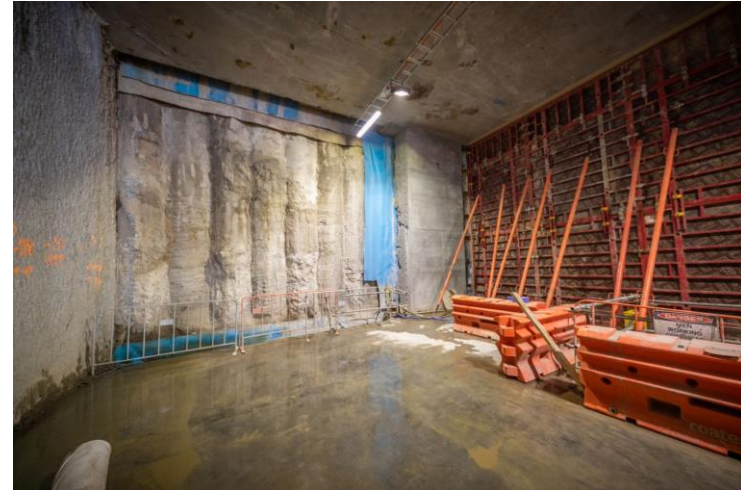
Eastbound tunnel entrance pile wall to be demolished
